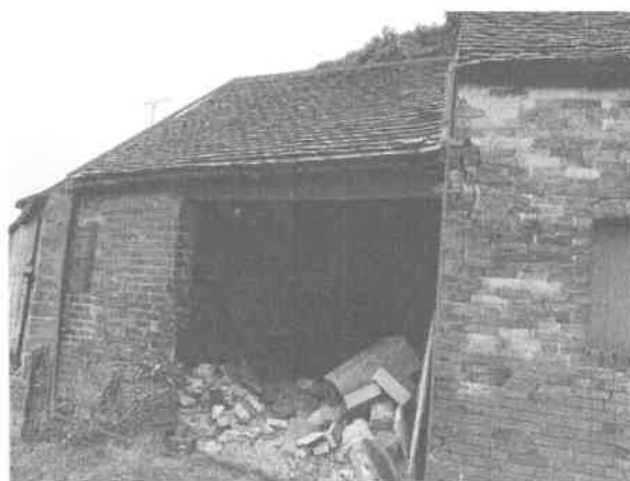
Image 3: North-west facing aspect of lean-to structure adjacent to Barn 2.
