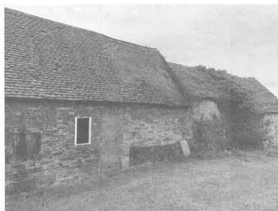
Image 4: South-east facing aspects of survey buildings.
