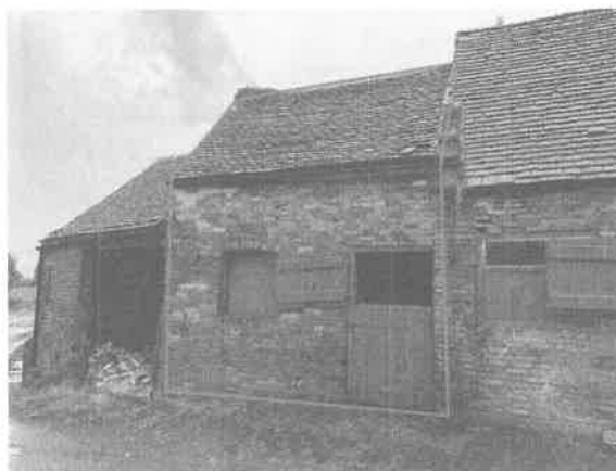
Image 2: North-west facing aspect of Barn
