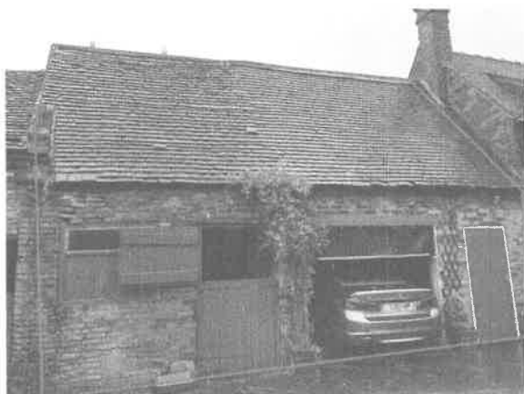
Image 1: North-west facing aspect of Barn 1. Note that that the building is subdivided. One half is used to park a motor vehicle (Section 1). Other us used by fan-tailed doves (Section 2)
