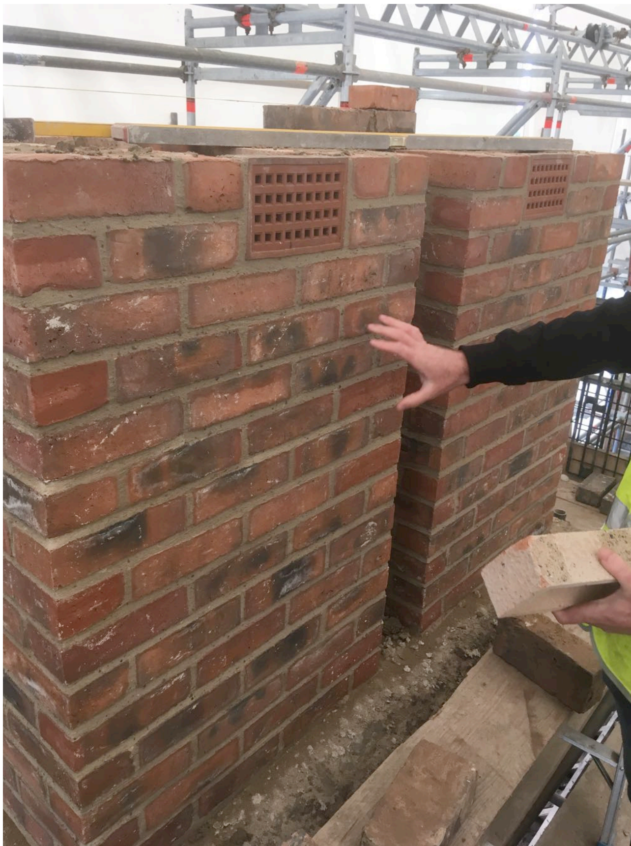
Installation of new air bricks to the rear of the rebuilt upper portion of chimney 6 – rebuilt from the level of the stone string course seen below.
