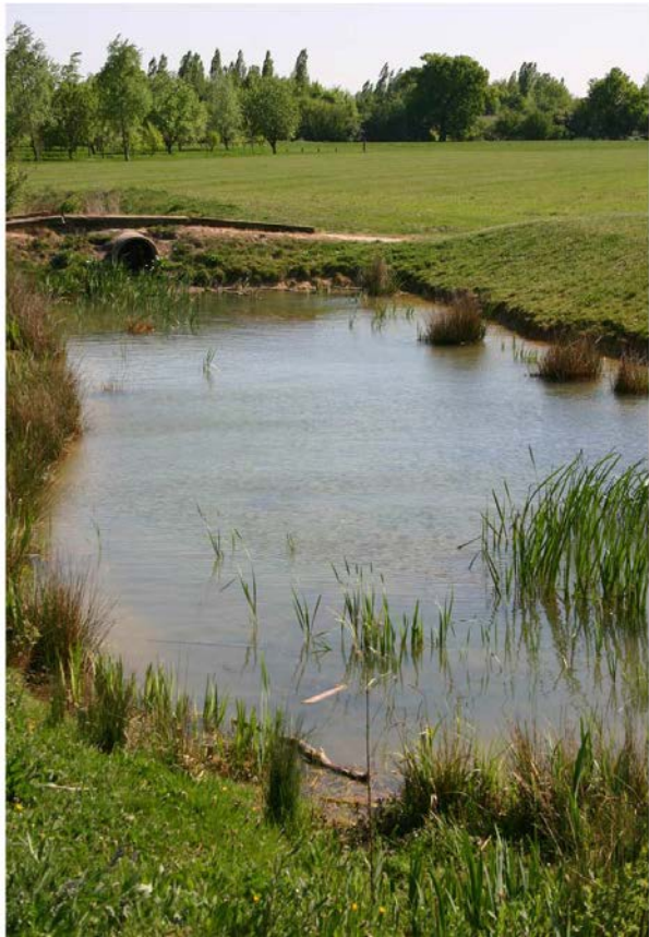
Integrated drainage and SUD's system
