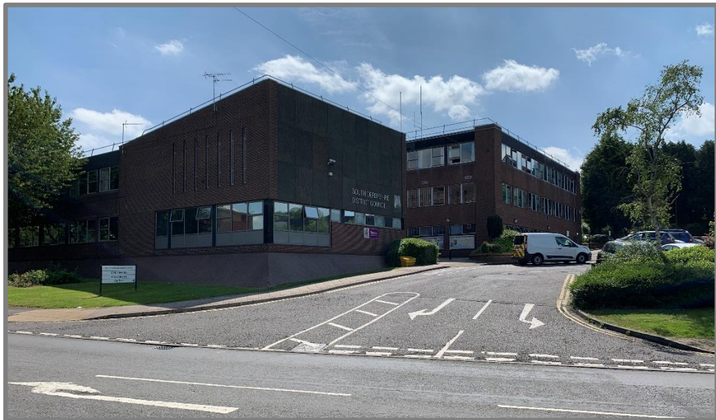
Fig 5 – South Derbyshire District Council Civic Offices on the adjacent side of the roundabout on William Nadin Way
