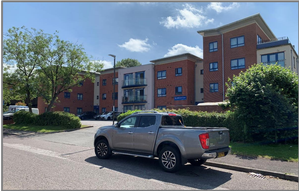
Fig 4 – Russell Aston Court – residential development on the adjacent side of Darklands Road, fronting onto Civic Way
