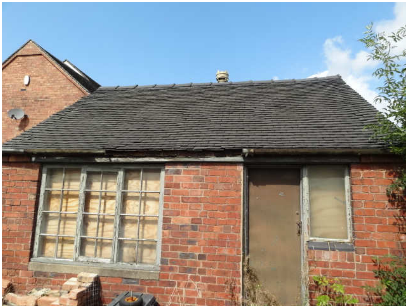
Photo showing building, from front, (looking north)
