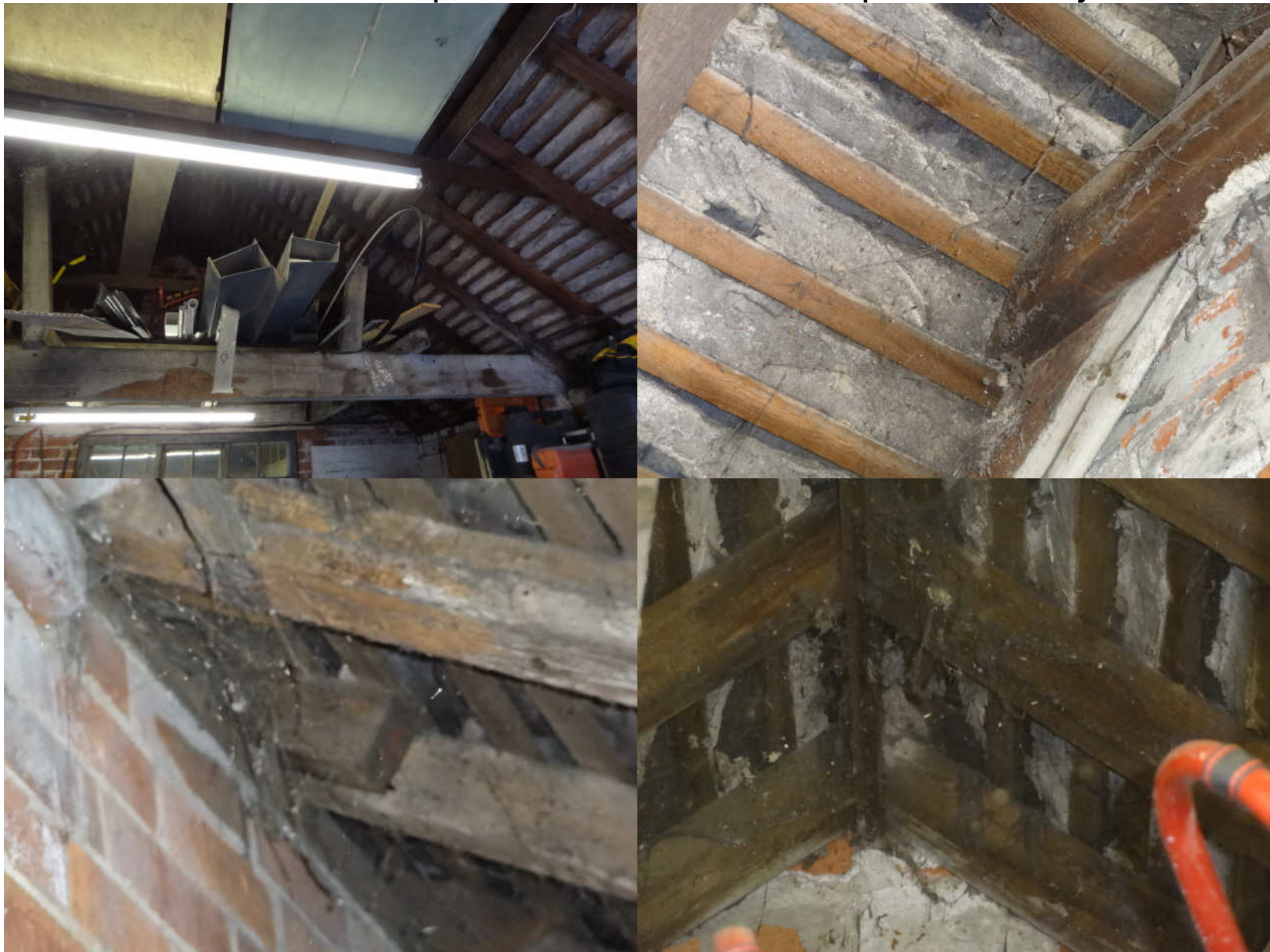
Photo showing roof timbers and spiders' webs in the roof space
