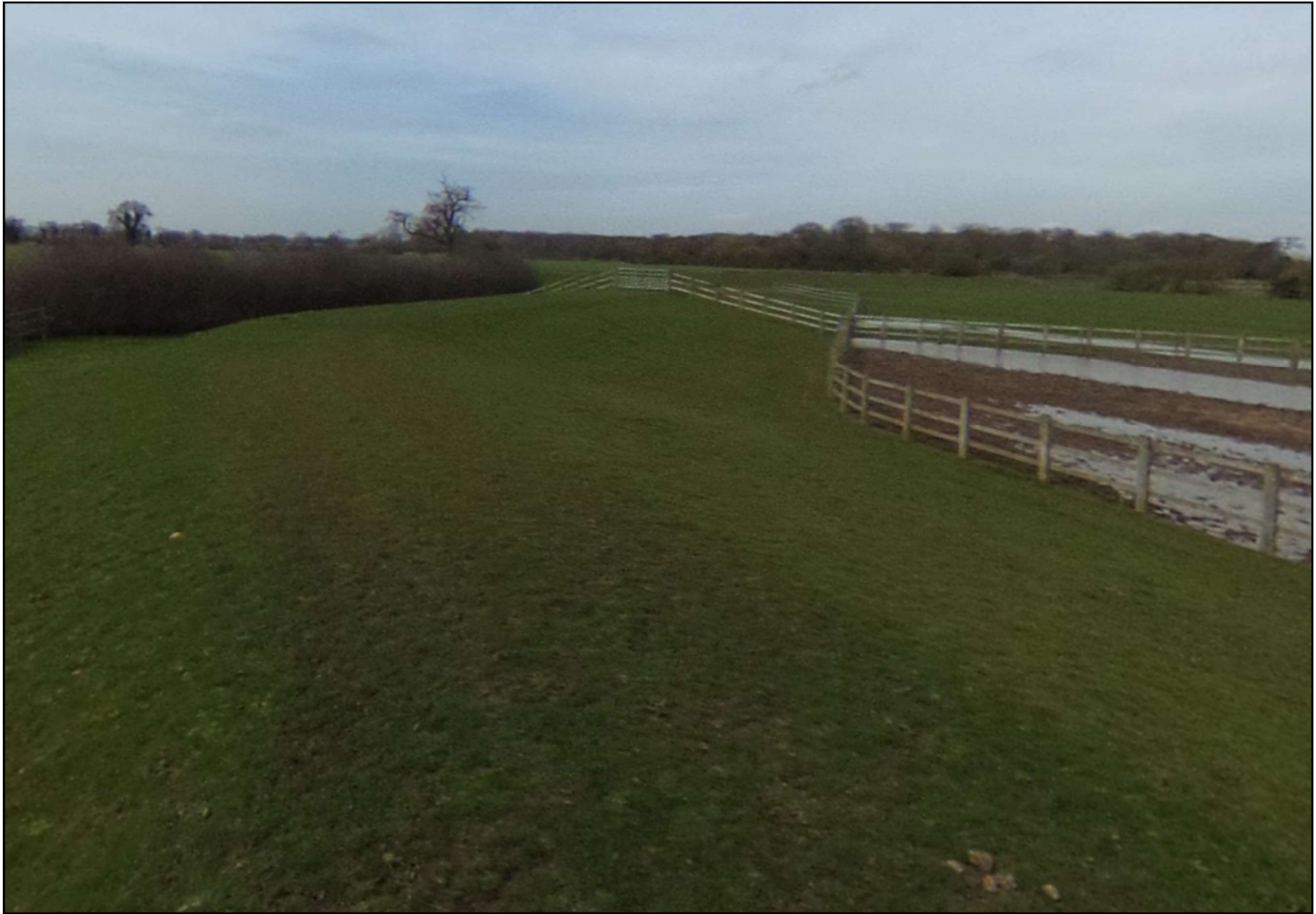
View looking north-west along earthen embankment, adjacent to Holme Farm Equestrian Centre.
