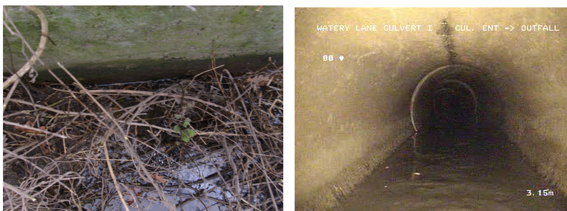
Figure 14 & 15: Picture illustrating condition of inlet and internal CCTV image of culvert spanning Watery Lane
