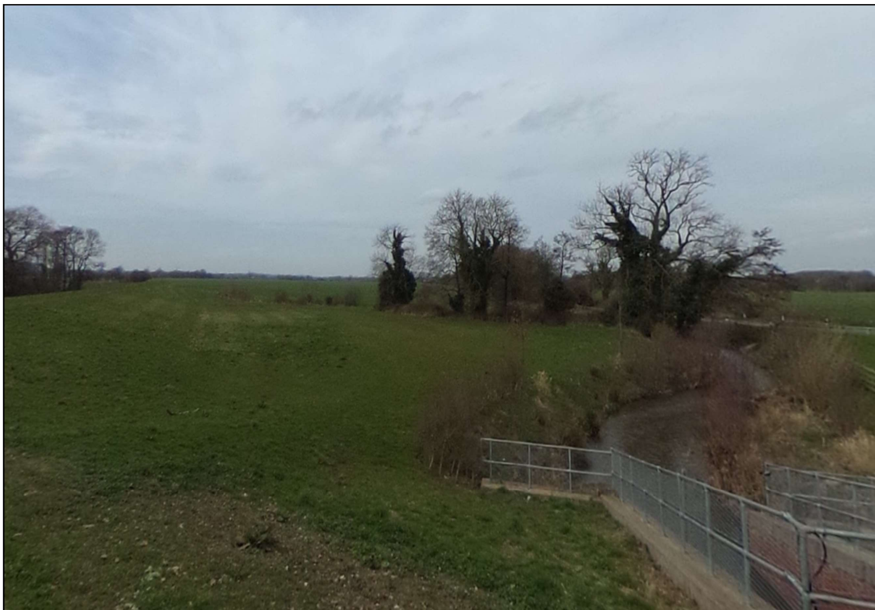
View looking westwards of the flood defences (L) on Brookside Farm across to the Foston Brook (R).
