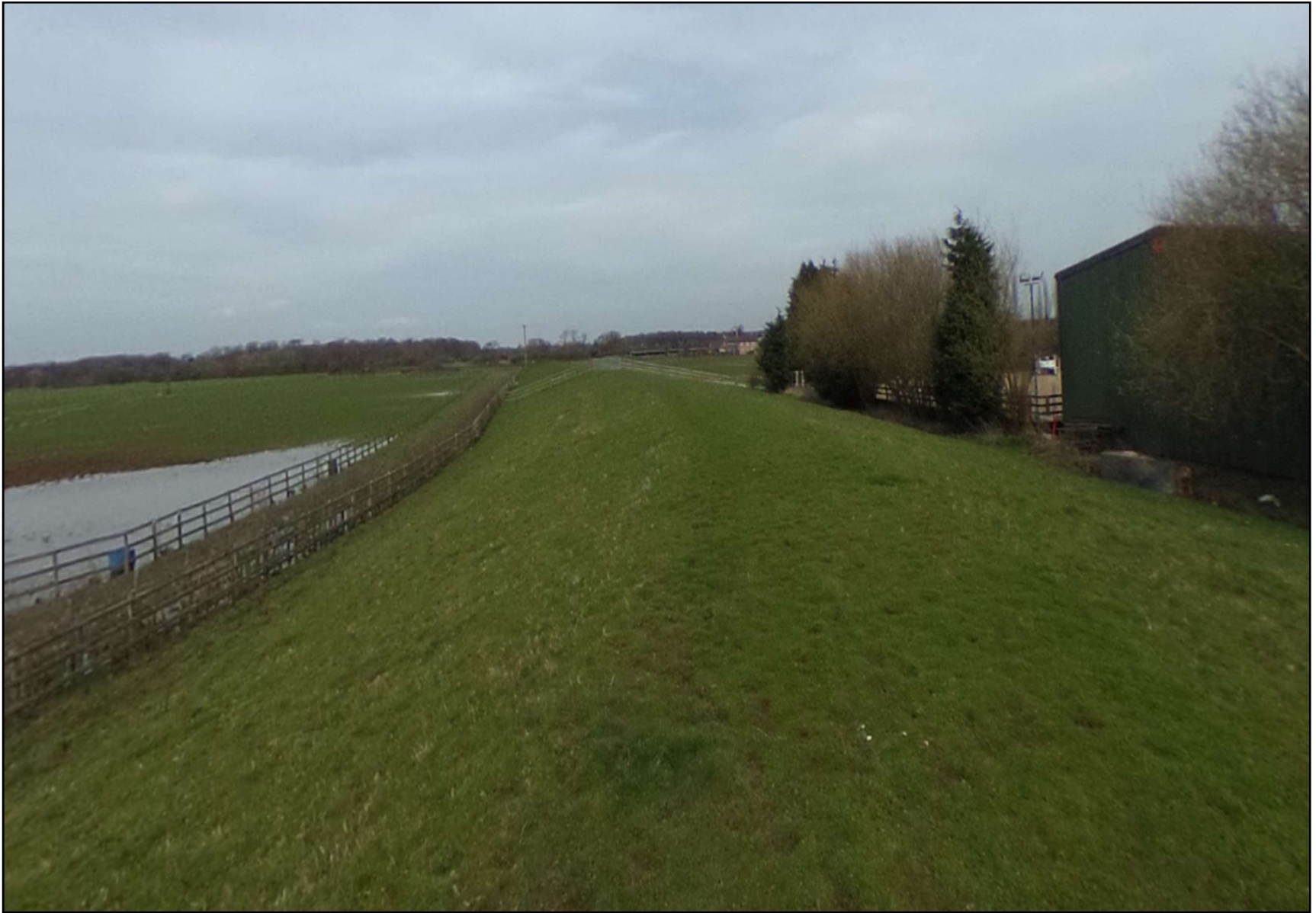
View looking northwards along earthen embankment, adjacent to Scropton Riding & Driving Centre.
