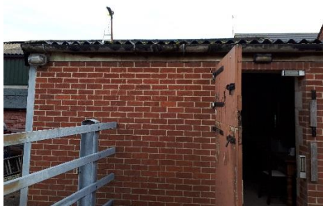
Photograph 7: Building B4 from west aspect
