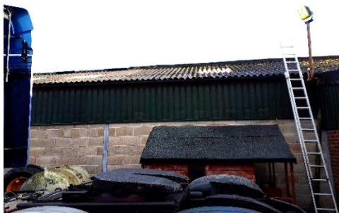
Photograph 5: Building B3 from west aspect
