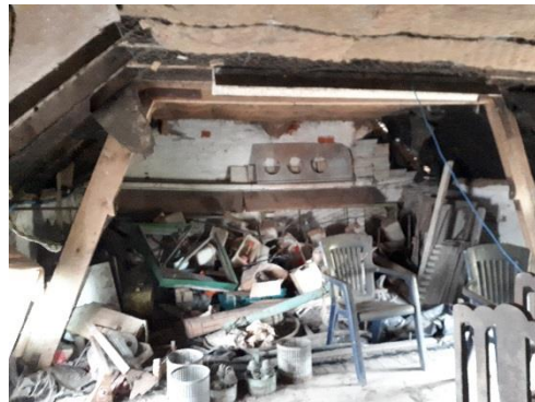
Photograph 10: Internal area of B5 (first floor)
