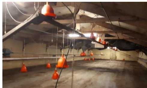
Photograph 2: Internal area of B1
