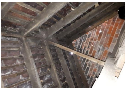
Photograph 11: Roof void in B5
