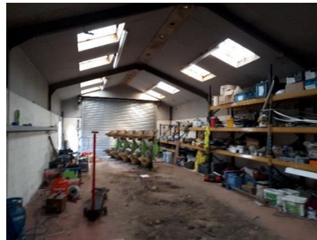
Photograph 6: Internal area of B3
