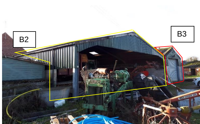
Photograph 4: B2 (yellow) and B3 (red) from north aspect
