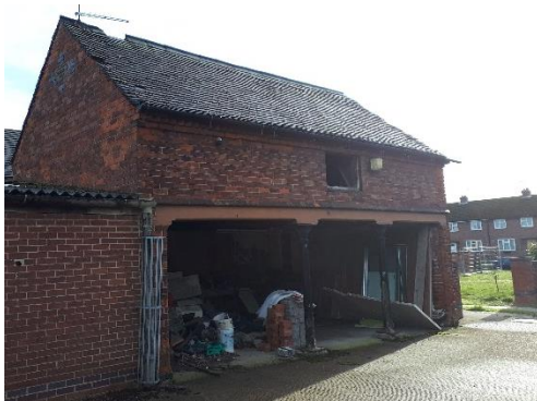
Photograph 9: Building B5 from west aspect
