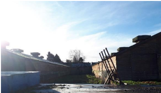
Photograph 1: Building B1 from northern aspect
