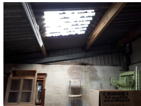
Photograph 8: Internal area of B4
