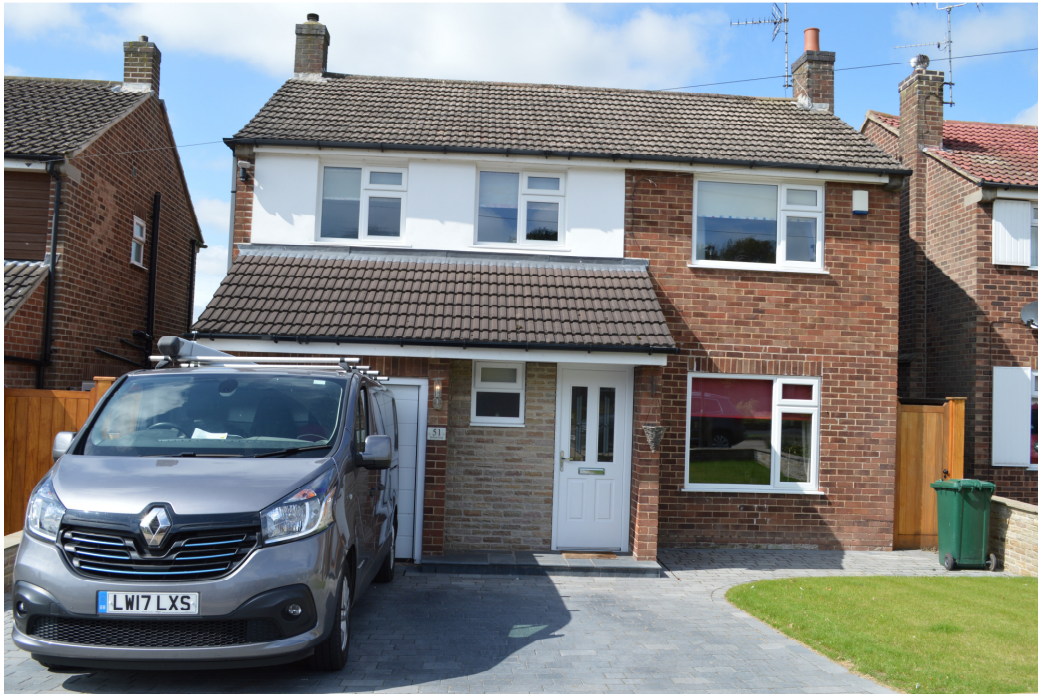
Front Elevation (east) of the existing house, which will remain unaltered.
