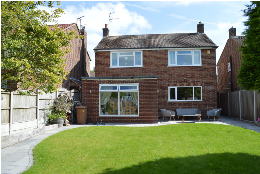
Rear (west) elevation, showing rear extension to be demolished
