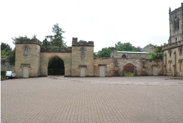
Fig. 07: The Gate houses (LHS) and hound enclosure form the boundary to the south side of the main castle yard. The west elevation of the Coach House is just visible in the RHS of the image. Image date Sept. 28 th 2014.
