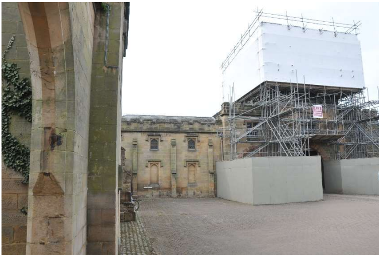
Fig. 04: View of the tented scaffold system around the clock tower erected in early 2016 to arrest the worst of the decay & to understand its structural issues. Image date April 11 th 2016.
