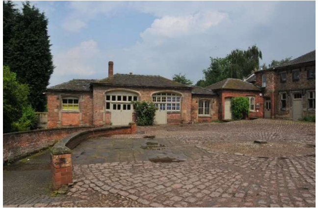
Fig. 10: The Grade II Listed Carriage Wash within the cobbled courtyard & north range of the Coach House. Image date June 9 th 2014.
