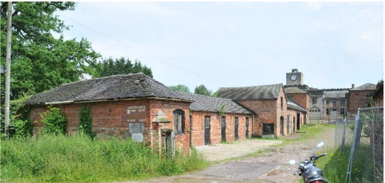
Fig. 11: Further afield, from the south west and looking through Lower Stable Yard, the Clock Tower structure is a relatively dominant feature of the Elvaston Castle estate. Image date June 9 th 2014.
