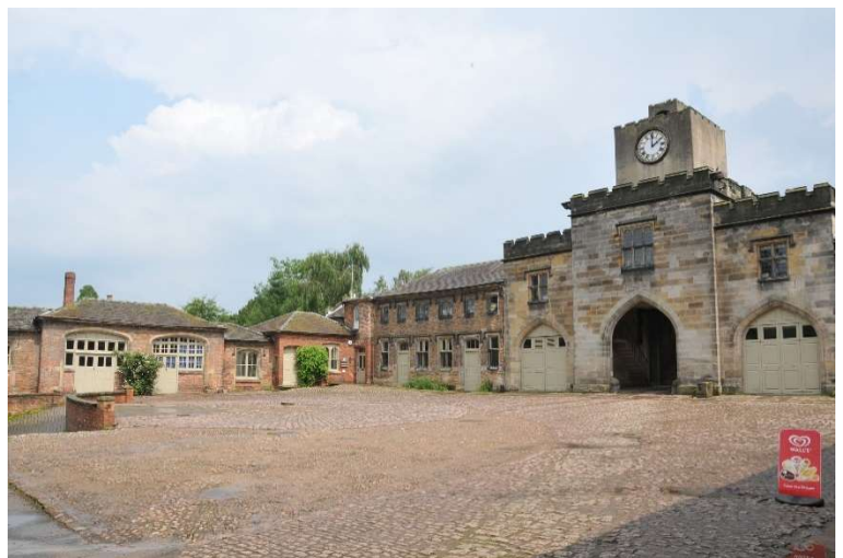
Fig. 01: View from south west corner of cobbled courtyard of single-storey north range and two-storey east range with clock tower above central open archway. Image date June 9th 2014
