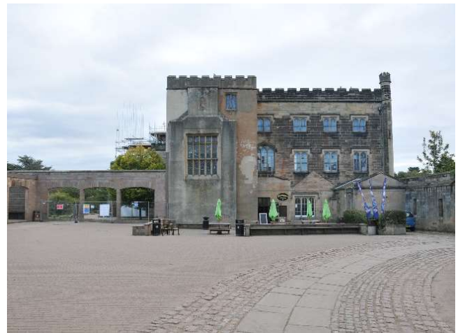
Fig. 06: The west elevation of the Main Castle building, adjacent to the Coach House, is less architecturally refined with a more utilitarian appearance, reflected by the function of the Main Castle Yard it overlooks. Image date Sept. 28 th 2014.
