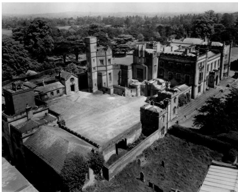
Fig. 15: Aerial view of castle courtyard looking north east showing the Coach House, the demolished north range and water tower, and Elvaston Castle. Image date c. 1920.
