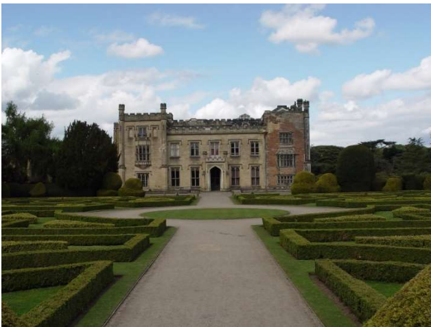
Fig. 05: The architectural purity & symmetry of south elevation of the main castle building is reflected in the layout of the decorative gardens of the GII RPG along the south avenue. Image date May 8 th 2013.
