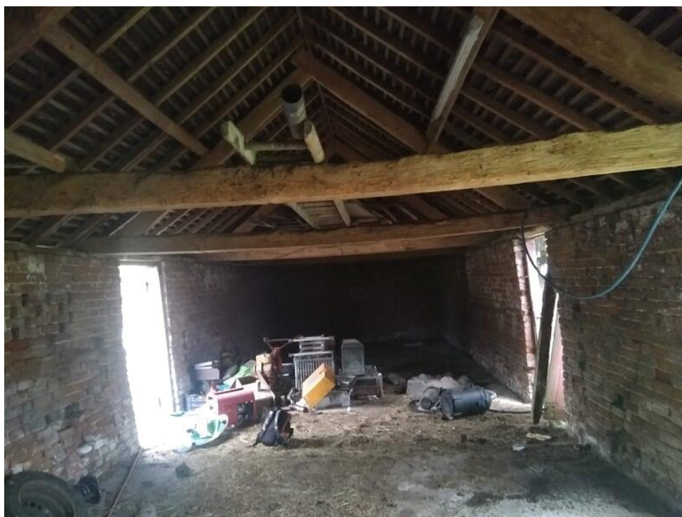
Plate 3: A photograph showing the internal space.
