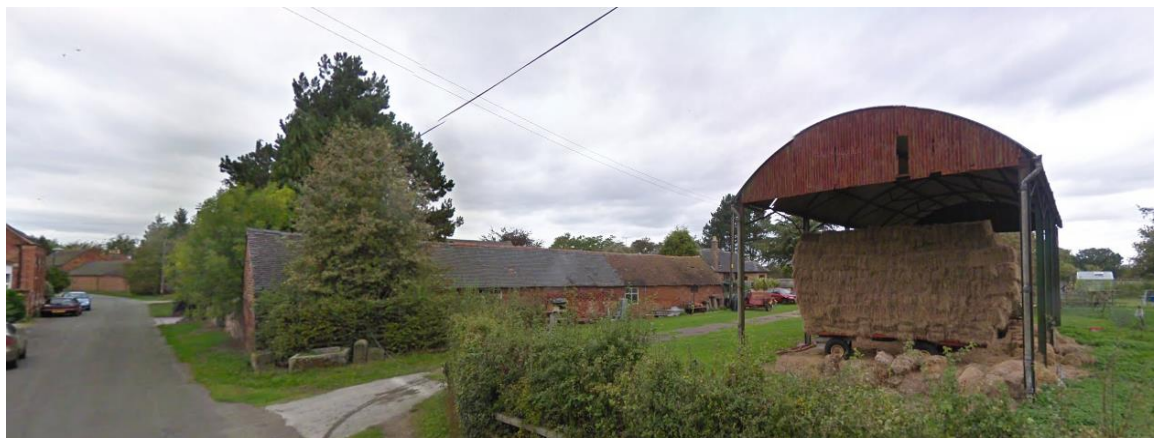
View looking west Duck Street showing existing barn & adjacent agricultural structure
