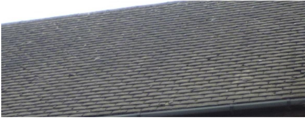
Existing roof tiles
