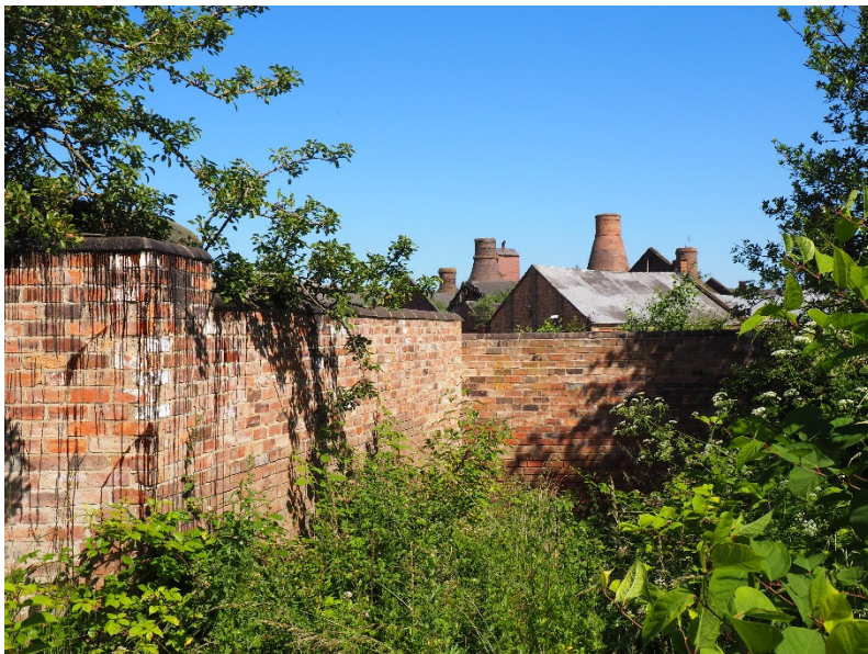
Plate 5: View eastwards from John Street towards Grade II* Green's Pottery bottle kilns
