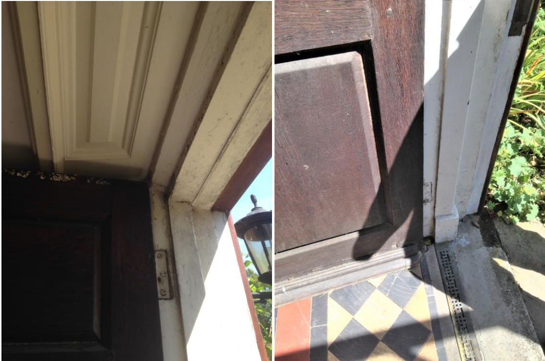
Figure 11 Internal door GD.19, frame and panelling with external door ED.02 in front. July 2019
