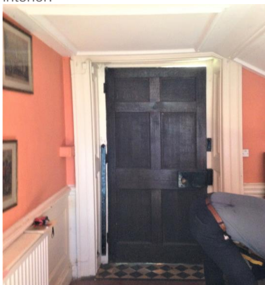
Figure 10 GD.19 in rear hallway shown closed, exterior door ED.02 is positioned behind, July 2019
