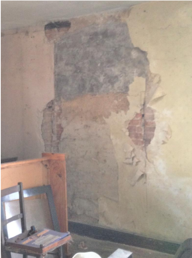
Figure 16 SW.12 External view and internal view showing straight joints, July 2019
