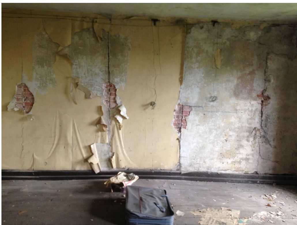
Figure 13 Straight joints visible at second floor (SW.08 and SW.09) July 2019
