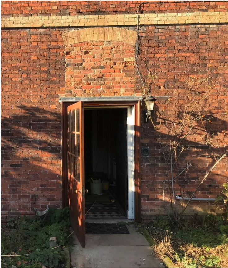
Figure 2 Existing external door ED.02 with existing white frame of internal door behind visible, July 2019
