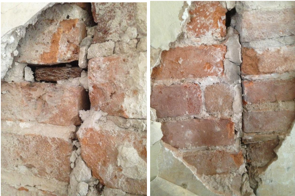
Figure 17 Straight joints between internal brick infill and adjacent masonry, with some timber visible (SW.12) July 2019
