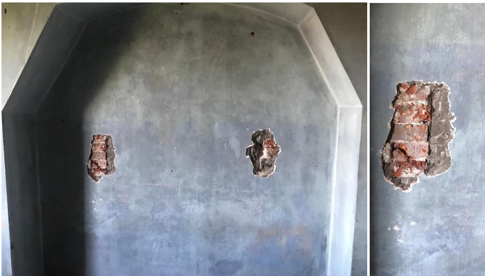
Figure 19 Straight joints visible internally (SW.24), Jan 2019
