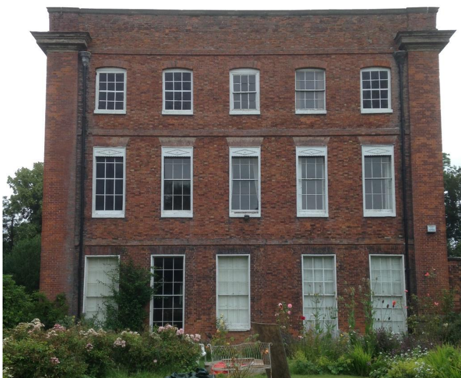
Figure 6 External view showing windows SW.08, SW.09 and SW.12 in context, July 2019
