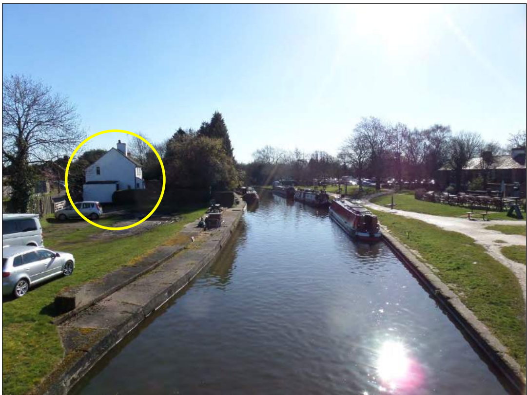
Photo 14 Cottage on north bank of the canal at Findern Lane
