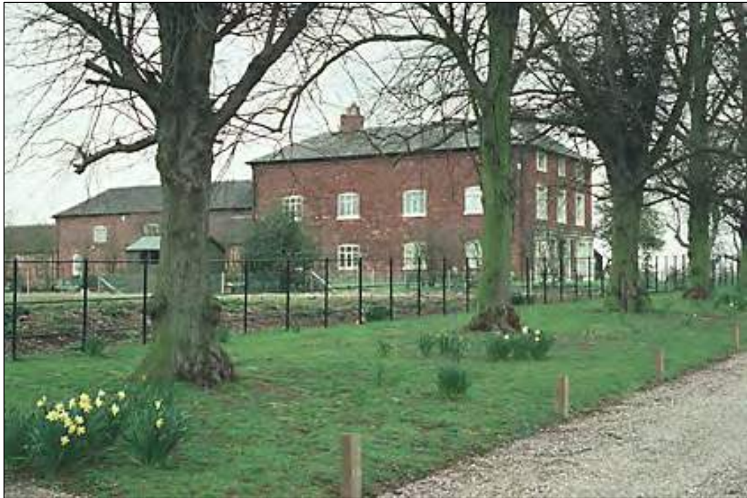
Photo 1a Willington Hill Farmhouse, viewed from the avenue (2004) (Image courtesy of Historic England – Images of England)
