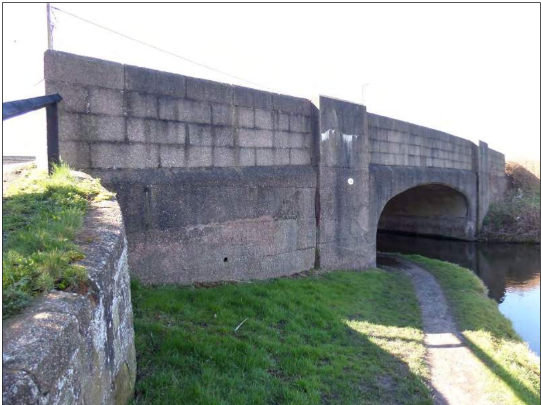
Photo 12 Modern concrete bridge of the A5132
