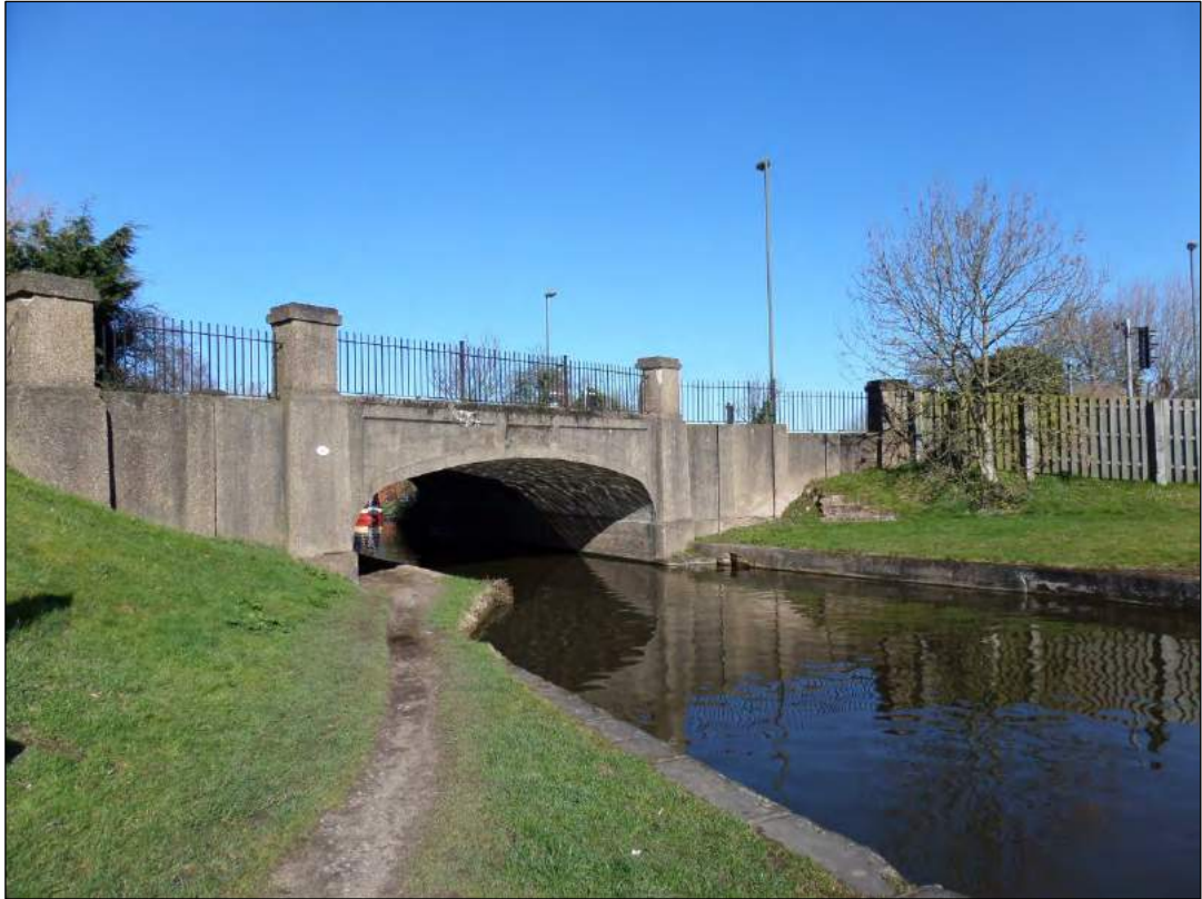
Photo 11 Modern concrete bridge of the B5008
