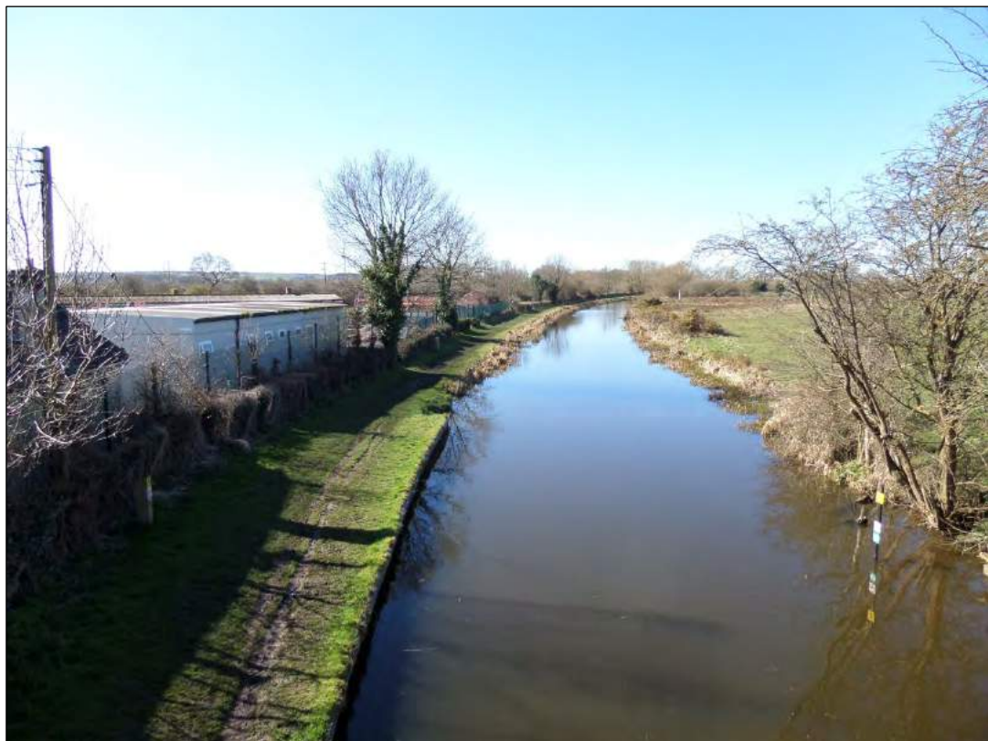
Photo 24 View south-west from the A5132 bridge
