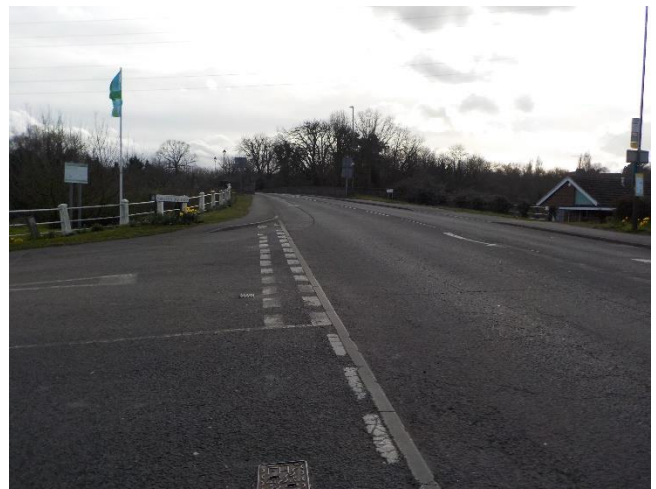
FIGURE 2: LOOKING SOUTH ALONG STATION ROAD
