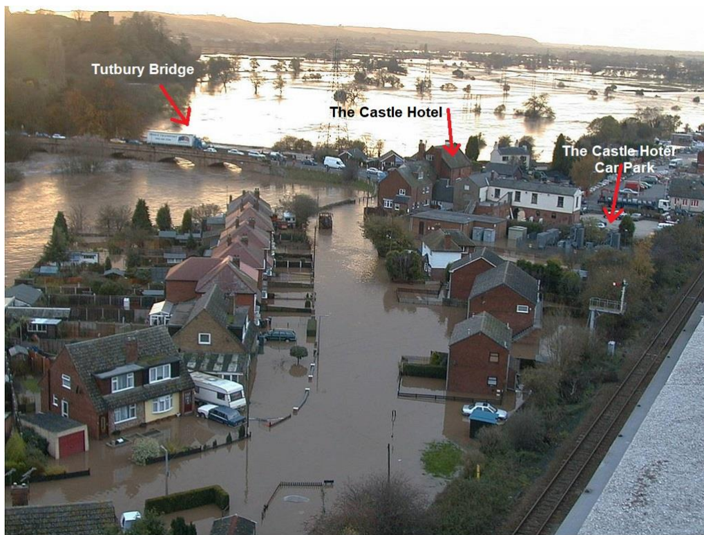
FIGURE 5: AERIAL VIEW OF TUTBURY BRIDGE AND THE CASTLE HOTEL DURING THE FLOOD IN 2000
