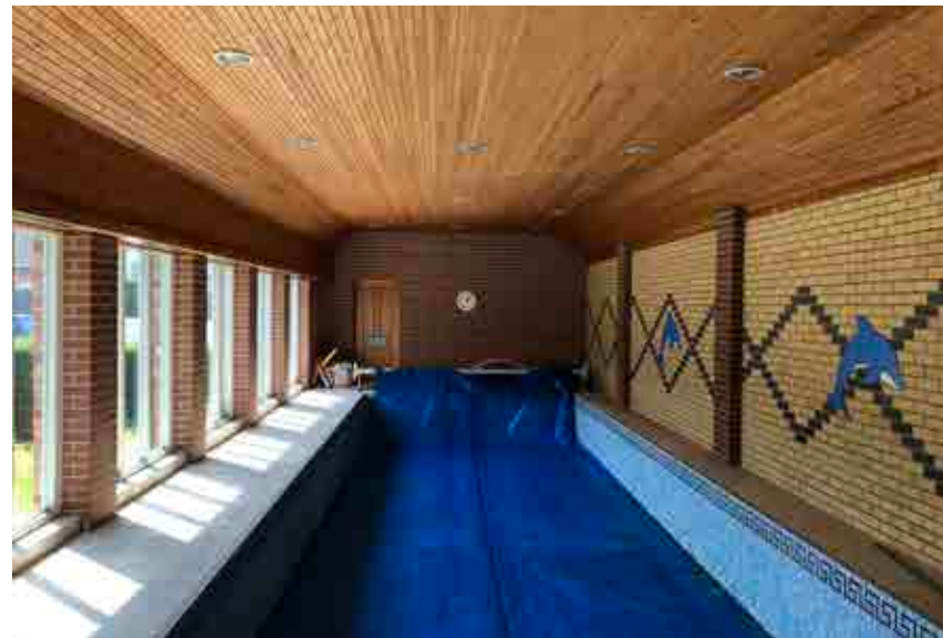
Existing swimming pool in west barn
