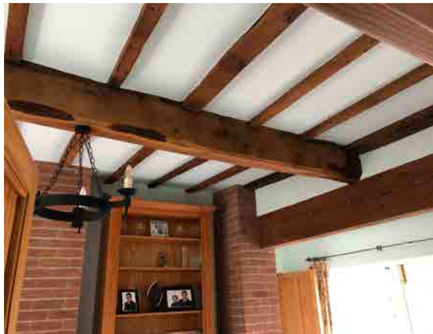
Exposed timber structure / beams within the existing dining room
