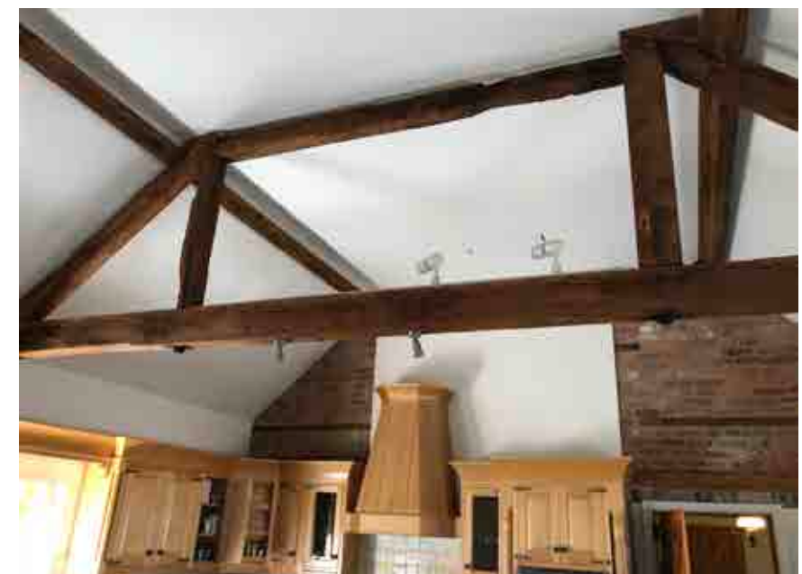
Timber truss and exposed purlins in the existing kitchen
