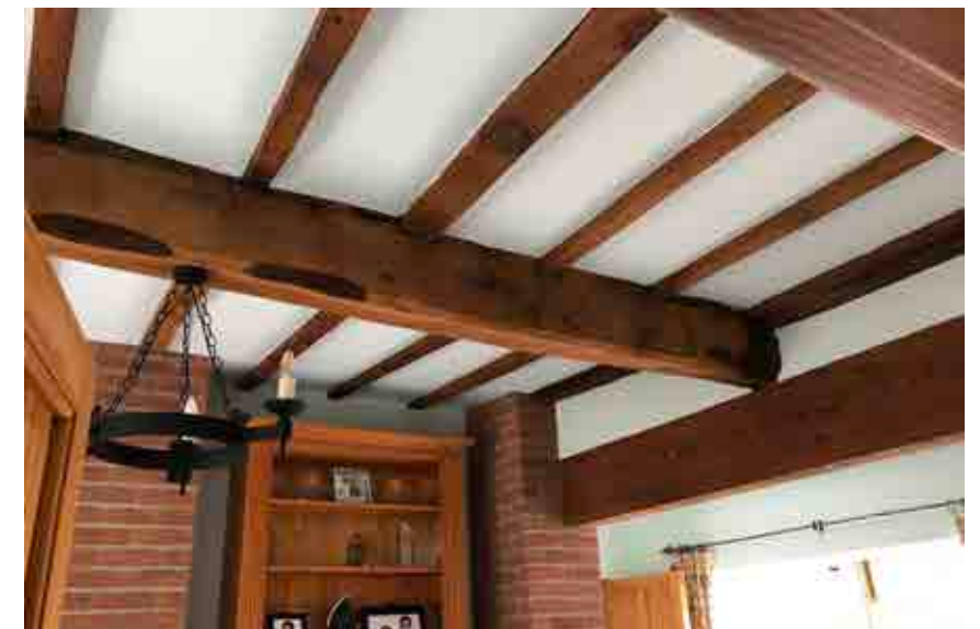
Retained historic features in existing dwelling (to become Unit 1)
