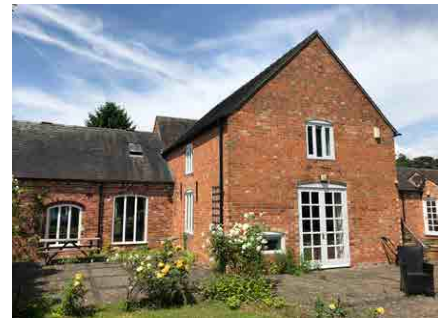
Brick detailing to rear east elevation
