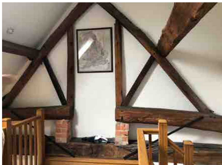
Exposed timber truss within landing
