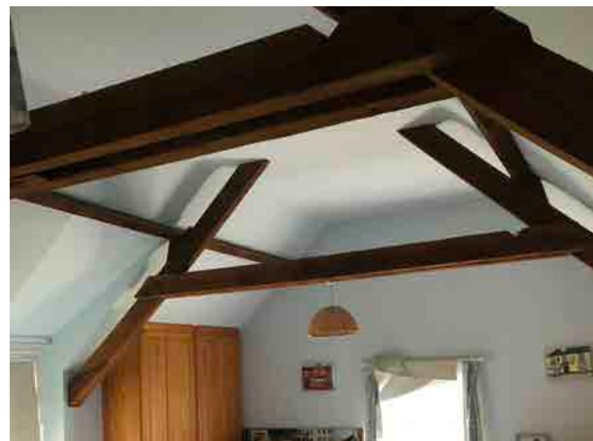
Timber trusses in the master bedroom
