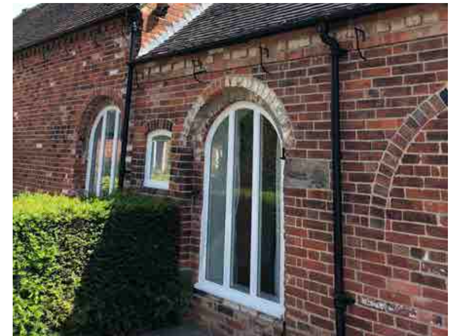
Brick and gutter detailing on eastern barn courtyard elevation
