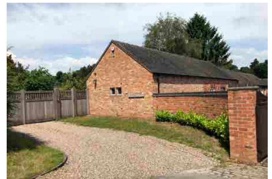
Access to adjacent Farmhouse and associated garage on site
