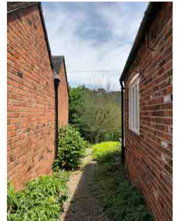
Existing pedestrian access to north gardens from courtyard
