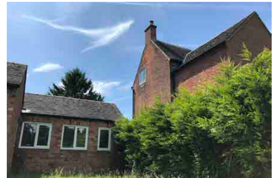
Proximity of north-west barn to neighbouring listed Farmhouse
