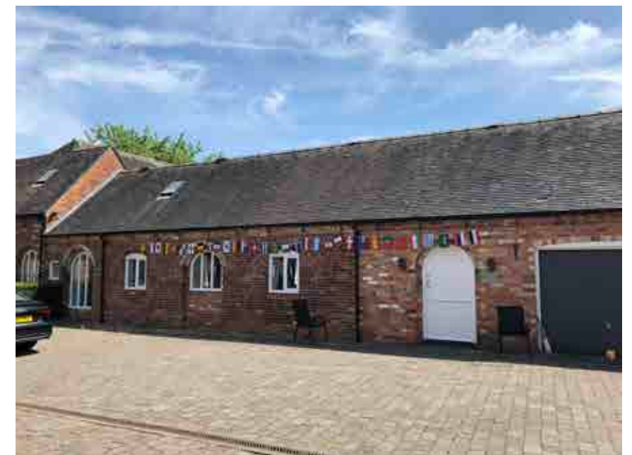
Evidence of previous extension and alteration to buildings
