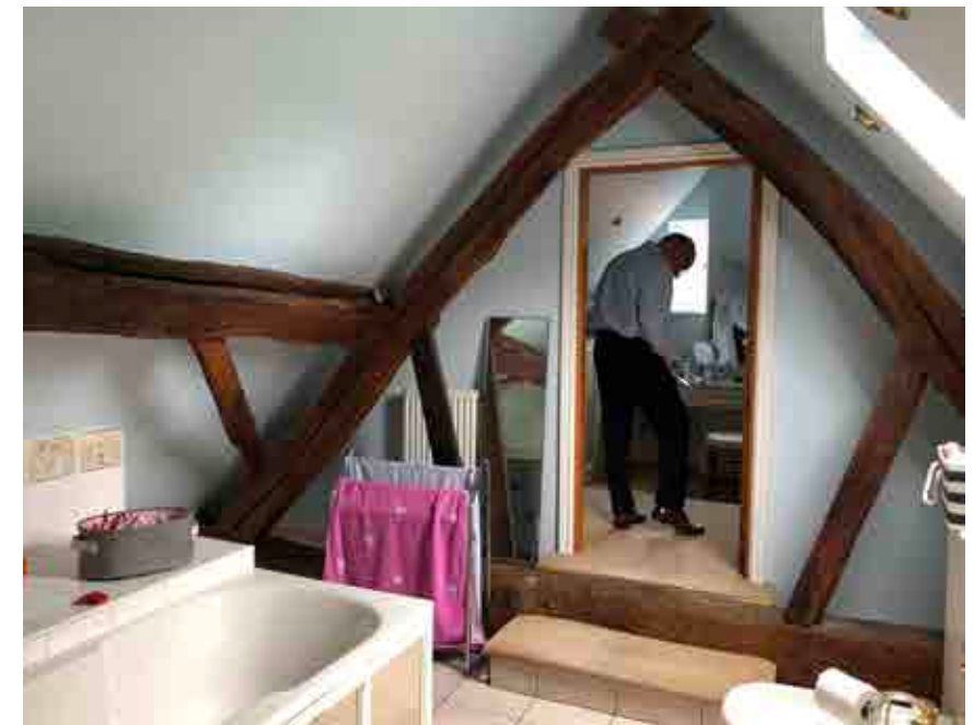
Timber truss and exposed purlins in the master bedroom ensuite
