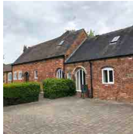
Existing courtyard paving
