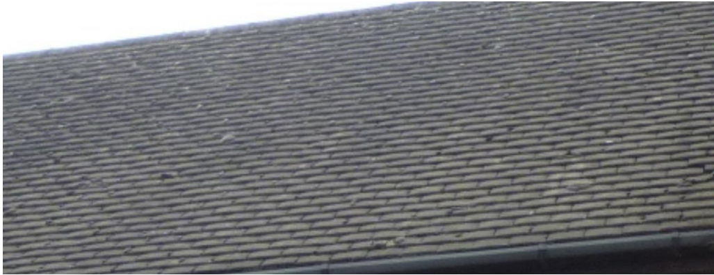
Existing roof tiles
