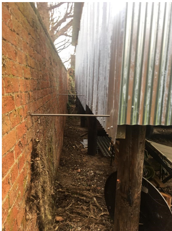
Photo 2 Tie bars through the store building
