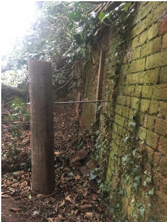
Photo 1 Supporting pole and tie-bar
