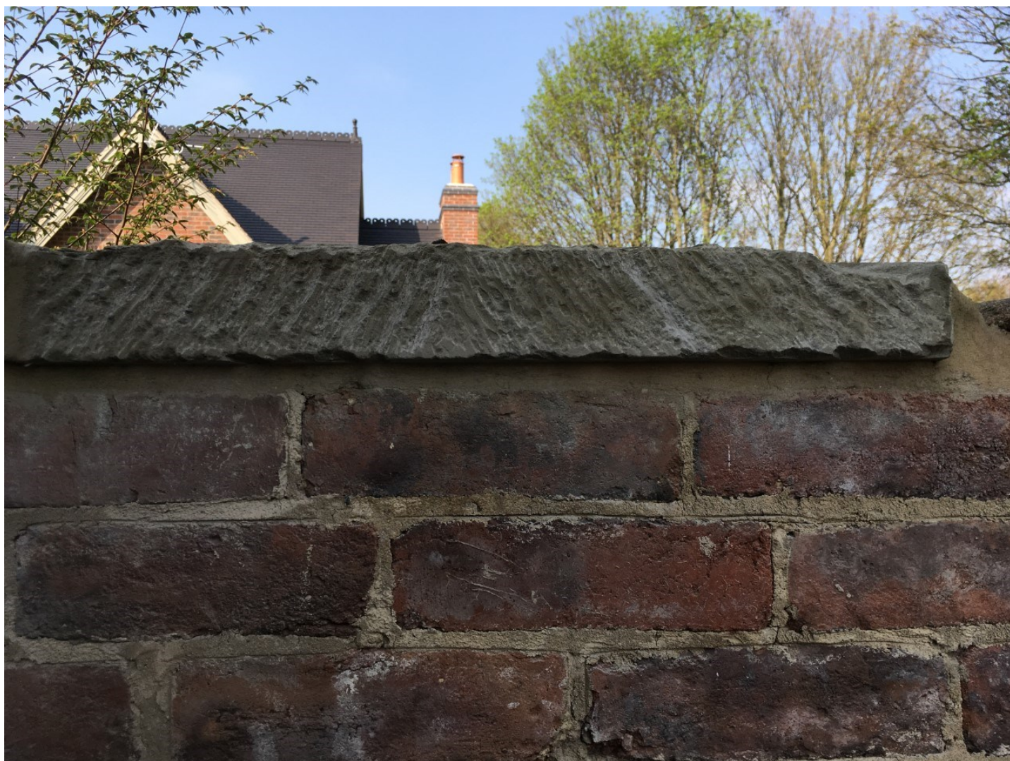
Photo 3—Capping stone showing tooling detail
