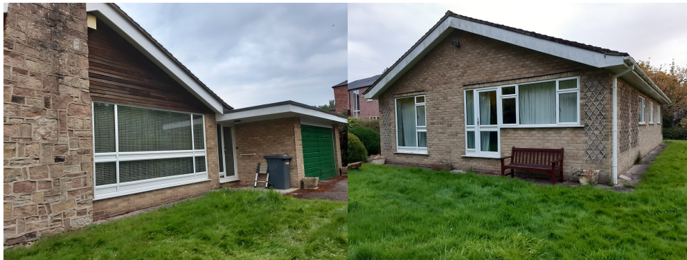
Photo: eastern and northern aspect of building B1 featuring attached garage, wooden boards and uPVC soffits
