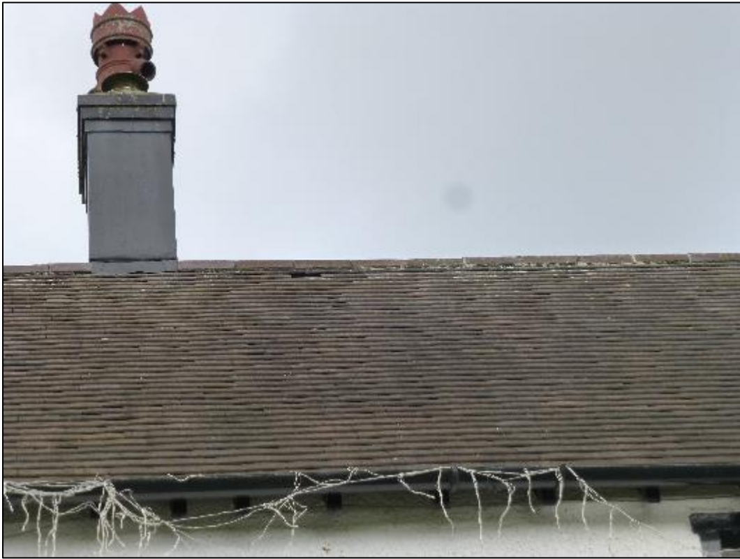
Photo 3. B1 – example access between tiles and lining
