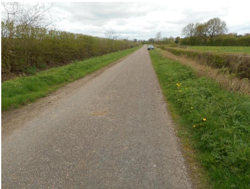
8. View along Green Lane, which forms the north-eastern boundary of the land
