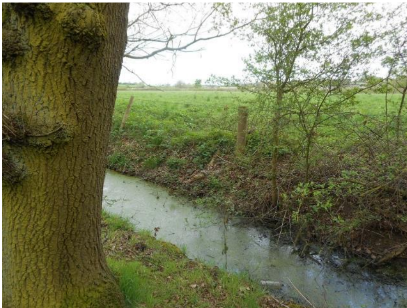
4. Water backing up in drainage ditch on boundary, which has been blamed on blockages in County Council land drains (action to alleviate blockages pending)
