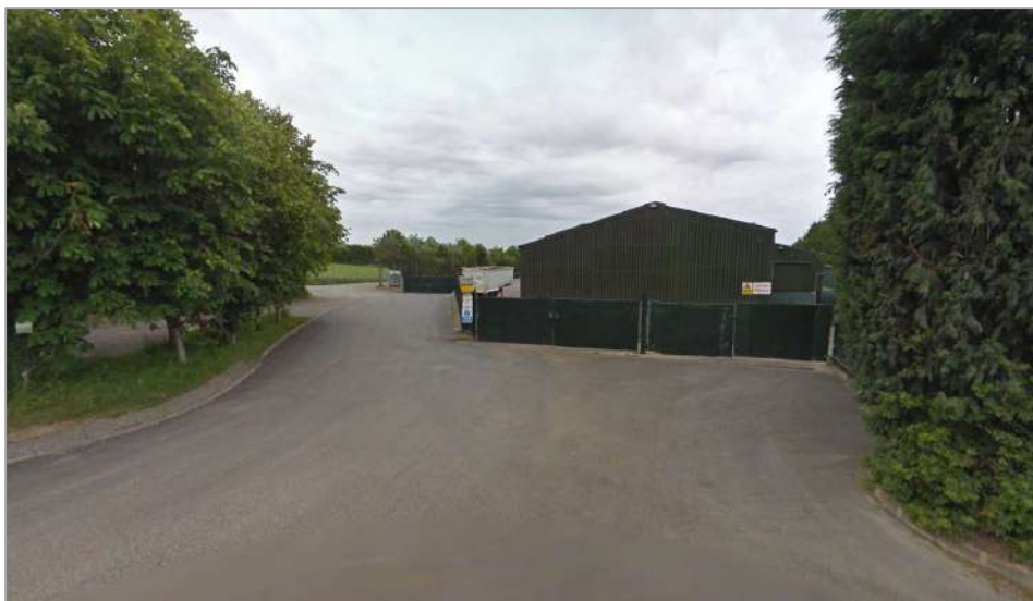
Original Frontage of the site @2011 Google Streetview showing the expanse of hardstanding
