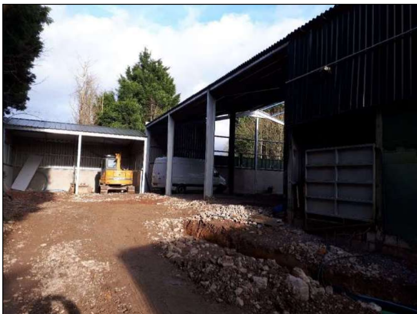
FIGURE 4.6 – New Water Tank Building prior to covered access extension being constructed:
