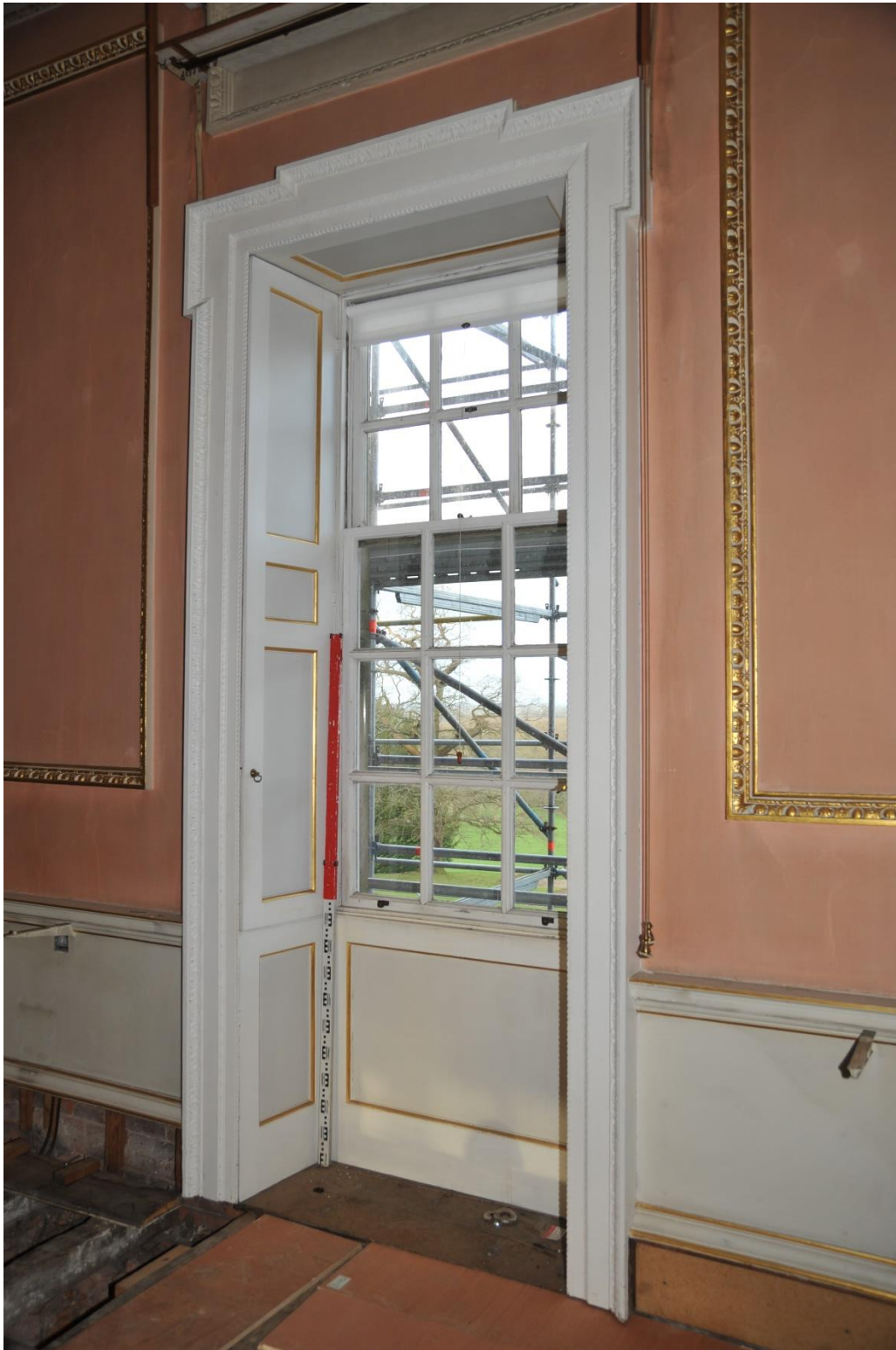
Pl.8: Inside of window reveal prior to work beginning, shutters open.
