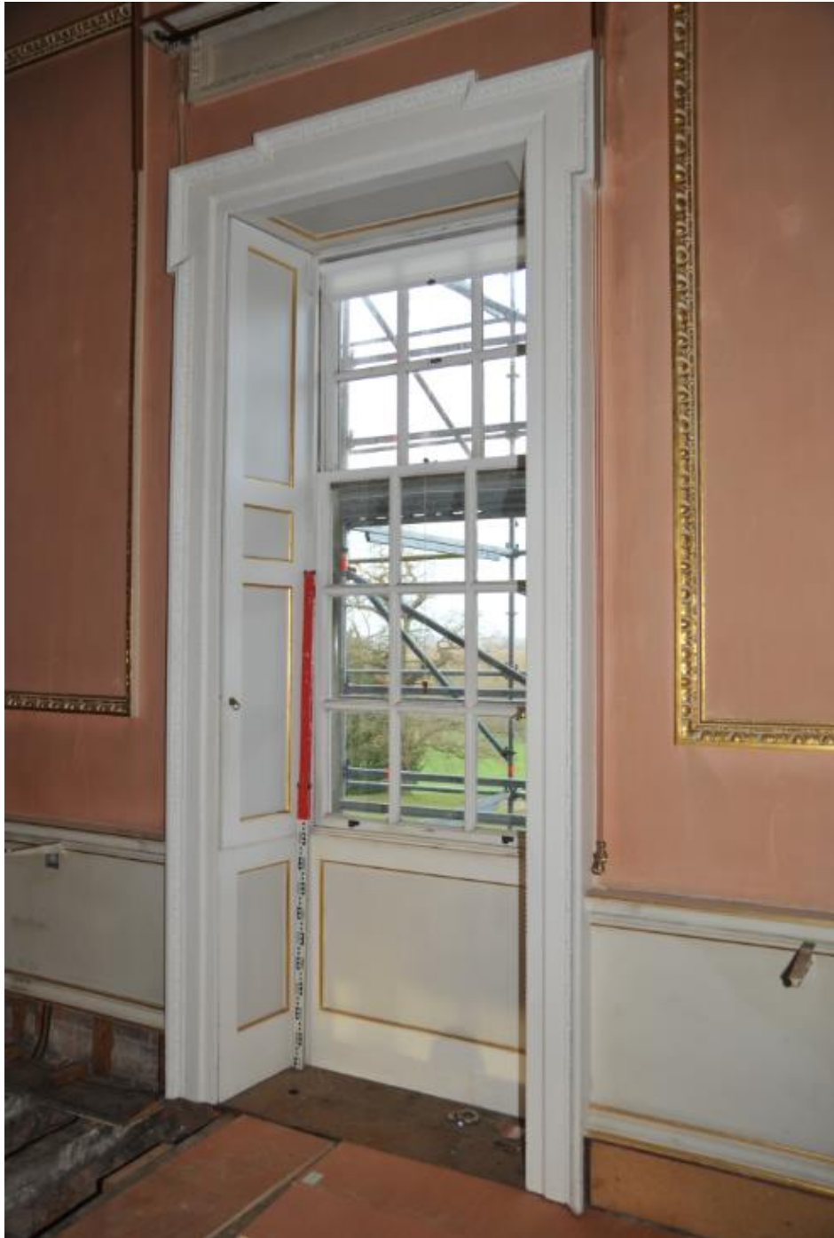
Pl.5: The reveal of the central window prior to works starting.
