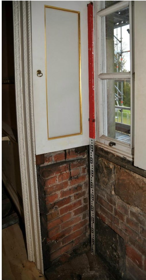
Pl.11: Northern side of reveal after removal of dado.
