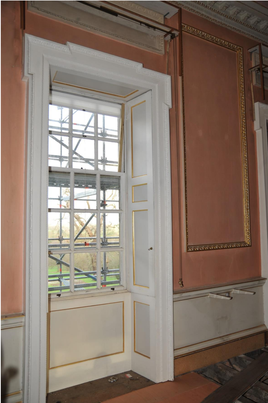
Pl.9: Inside of window reveal prior to work beginning, shutters open.
