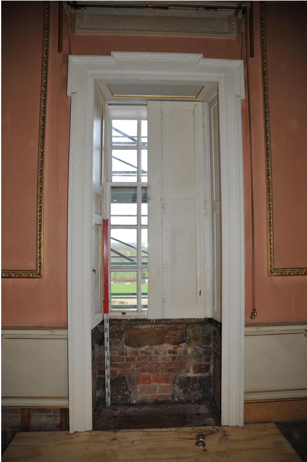
Pl.10: Inside of window reveal with dado panels removed.
