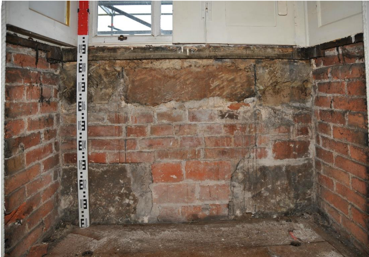
Pl.12: Detail of stone and brick masonry in reveal after dado removed.
