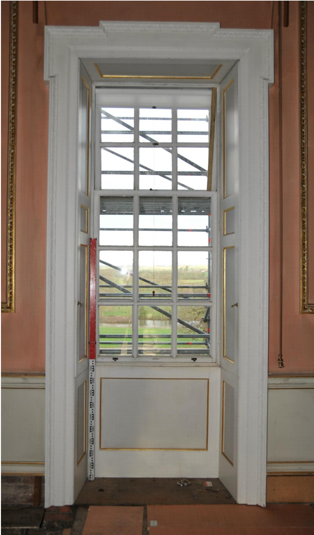
Pl.7: Inside of window reveal prior to work beginning, shutters open.
