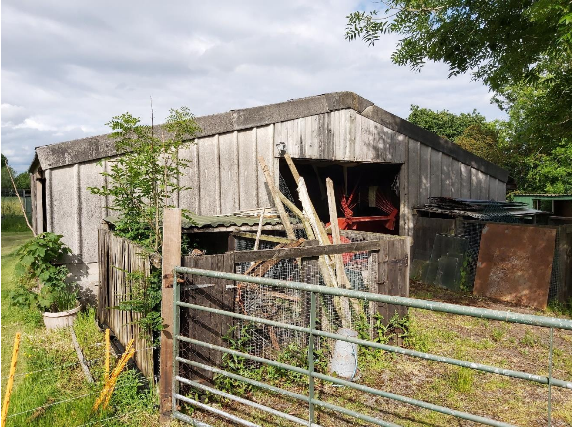
Figure 2 - Southwest elevation of building
