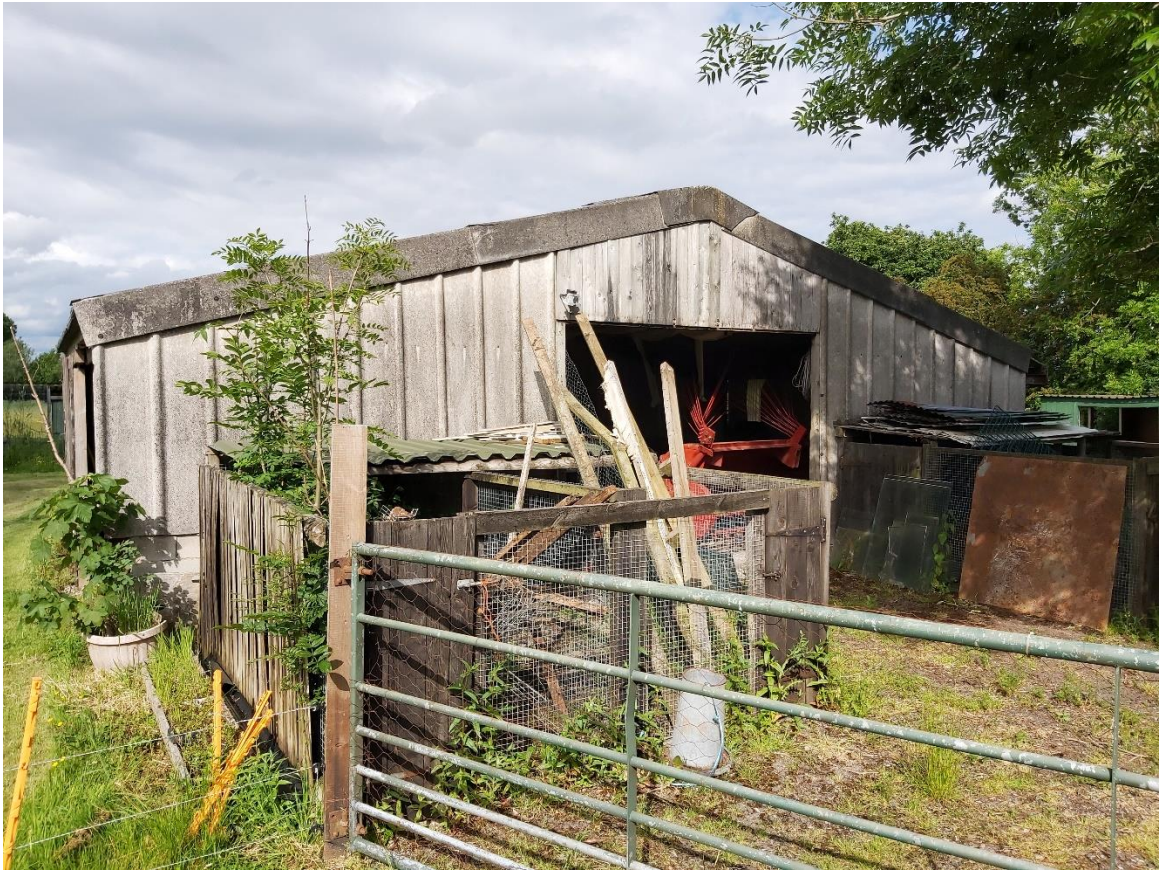
Figure 4 - Southwest elevation of building
