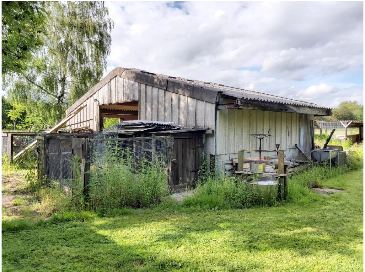
Figure 6 - The southwest (left) and southeast (right) elevations of the building
