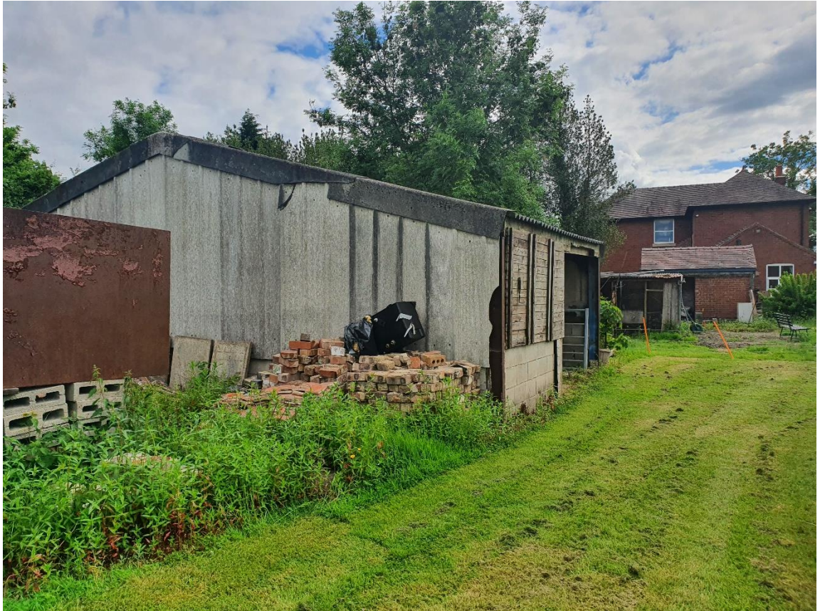
Figure 5 - The northeast (left) and northwest (right) elevations of the building. The dwelling can be seen in the right of the picture
