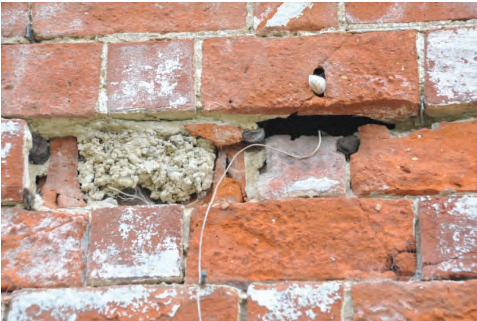
Fig. 13 (top): A substantial existing hole, of approx half a metre in length and 1-2 courses in depth, within the wall at a low level was sufficient to permit a camera to be inserted by hand to inspect its internal construction. The cast-iron heating pipe, running horizontally, is just visible at the bottom of the opening.
