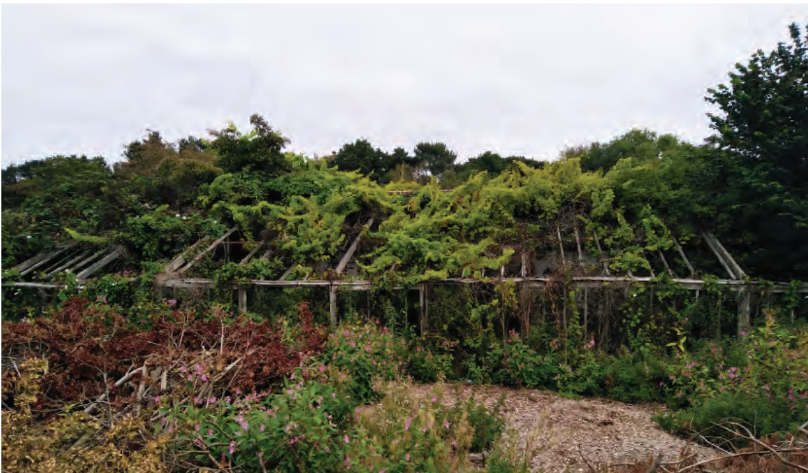
Fig. 26: Historic lean-to glasshouses remain on the south side of the south wall to the OEG.
