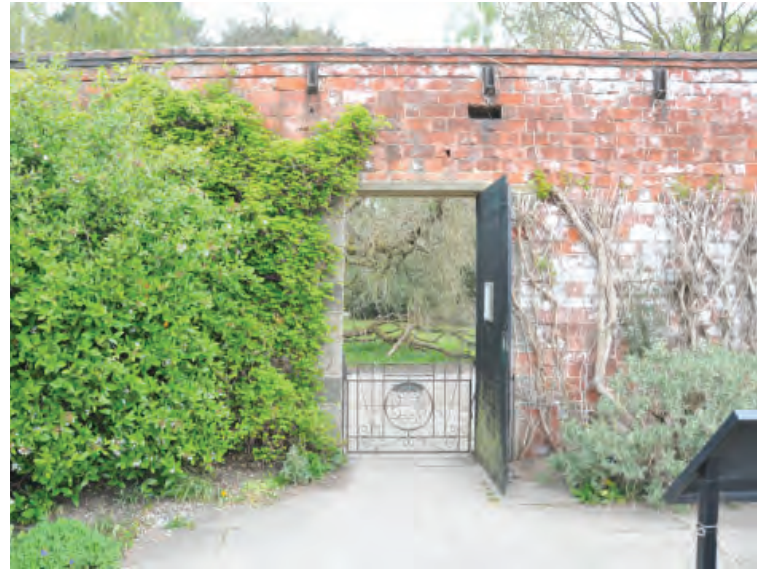
Fig. 5: Entrance from south side (interior) of the wall; the double gate arrangement is to be replaced with a single gate.
