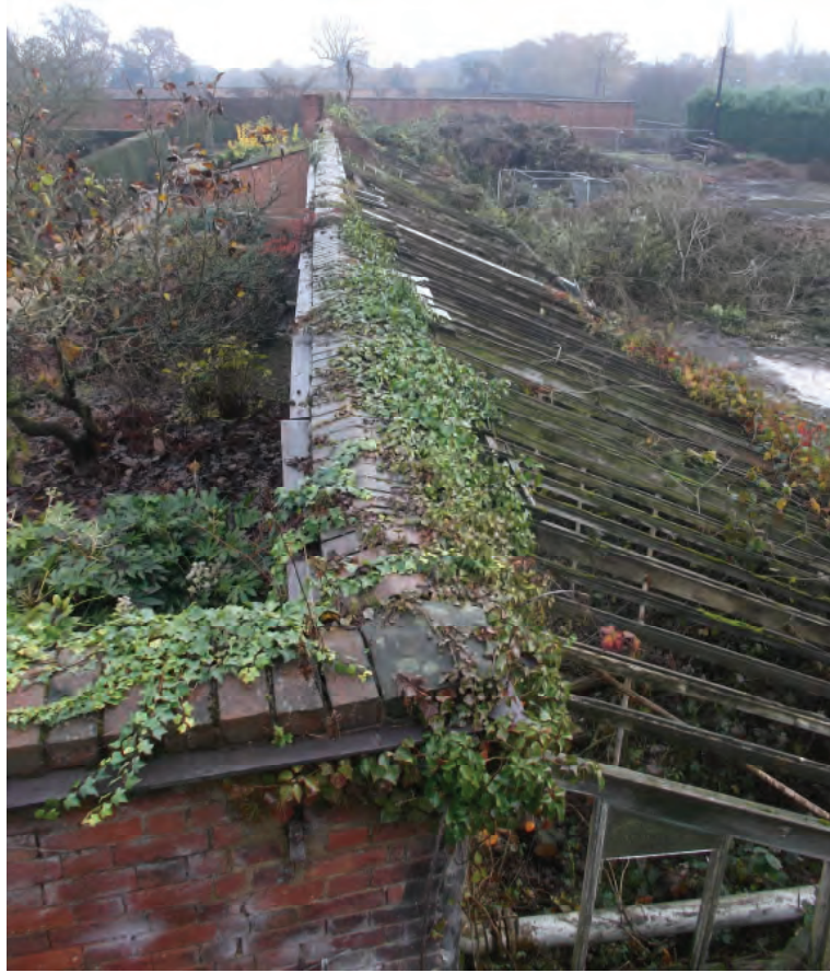
Photograph 5 - Wall D – view along top of wall.
