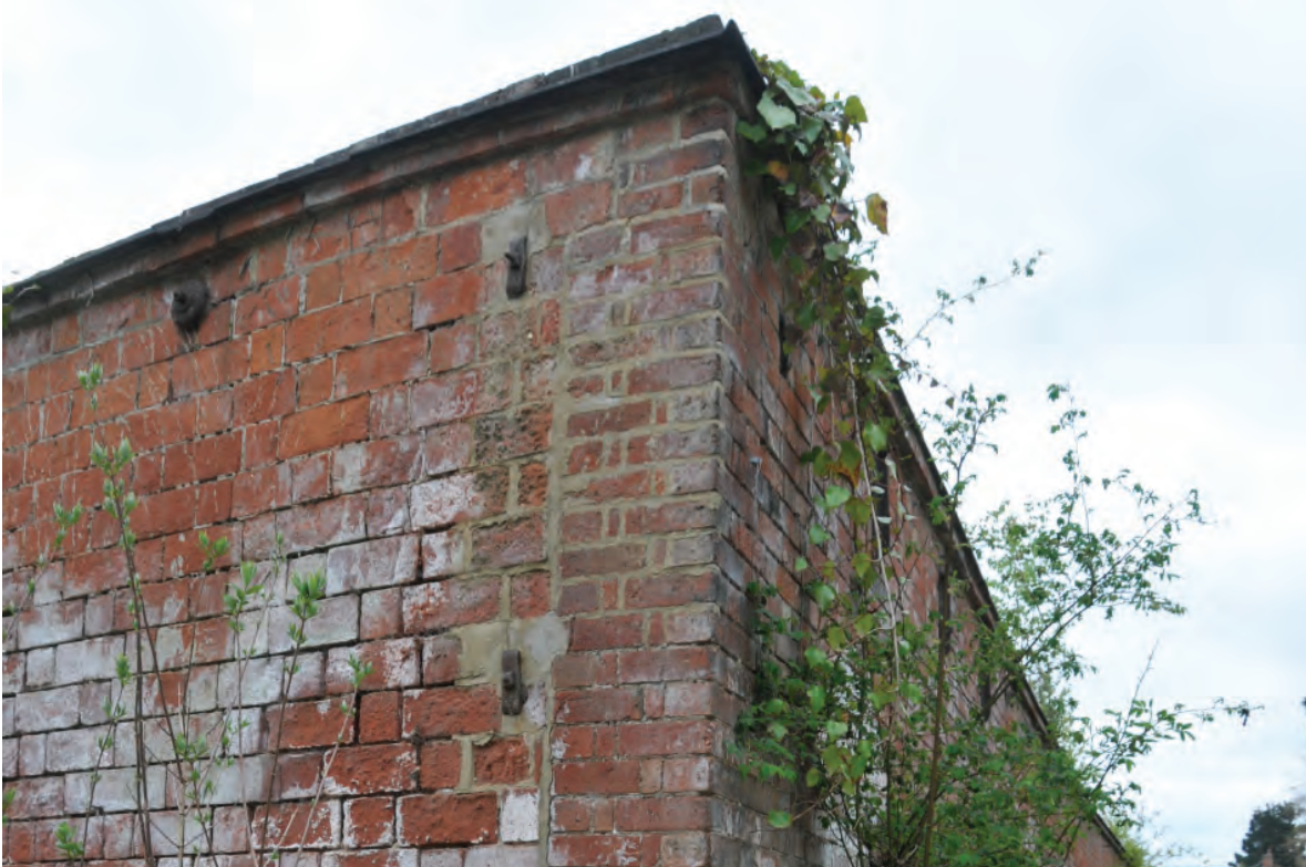
Fig. 27: A crude junction between the north heated wall and west wall of the OEG; notwithstanding the differing sizes in bricks these the adjoining structures simply abut each other rather than being toothed or properly tied together to ensure greater structural stability.
