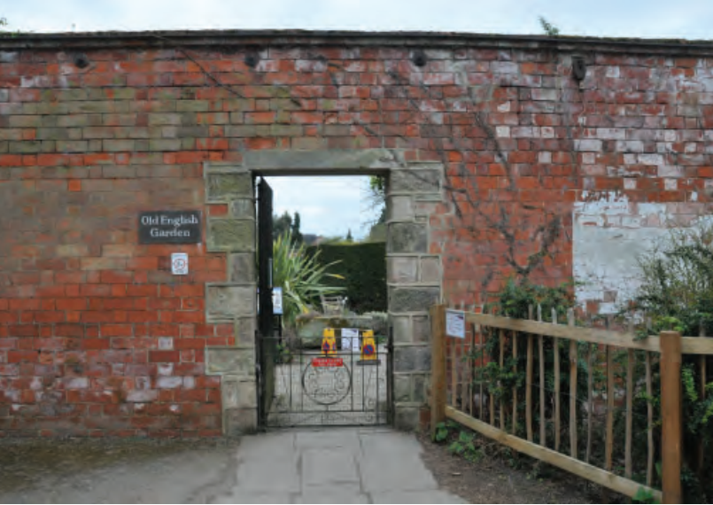
Fig. 4: Visitor entrance from north side (exterior) of the former heated garden wall; to be rebuilt to the same size.
