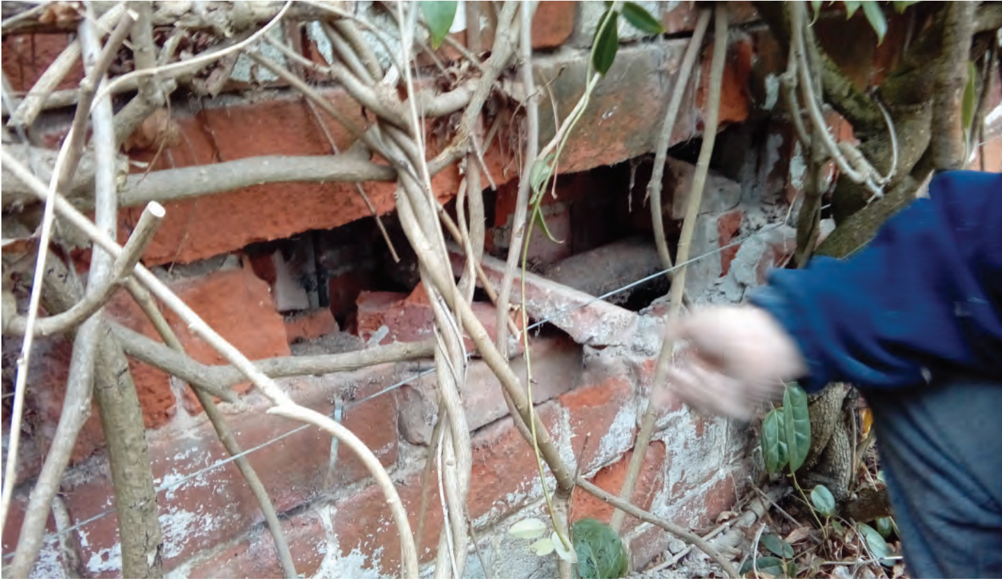
Fig. 13 (top): A substantial existing hole, of approx half a metre in length and 1-2 courses in depth, within the wall at a low level was sufficient to permit a camera to be inserted by hand to inspect its internal construction. The cast-iron heating pipe, running horizontally, is just visible at the bottom of the opening.
