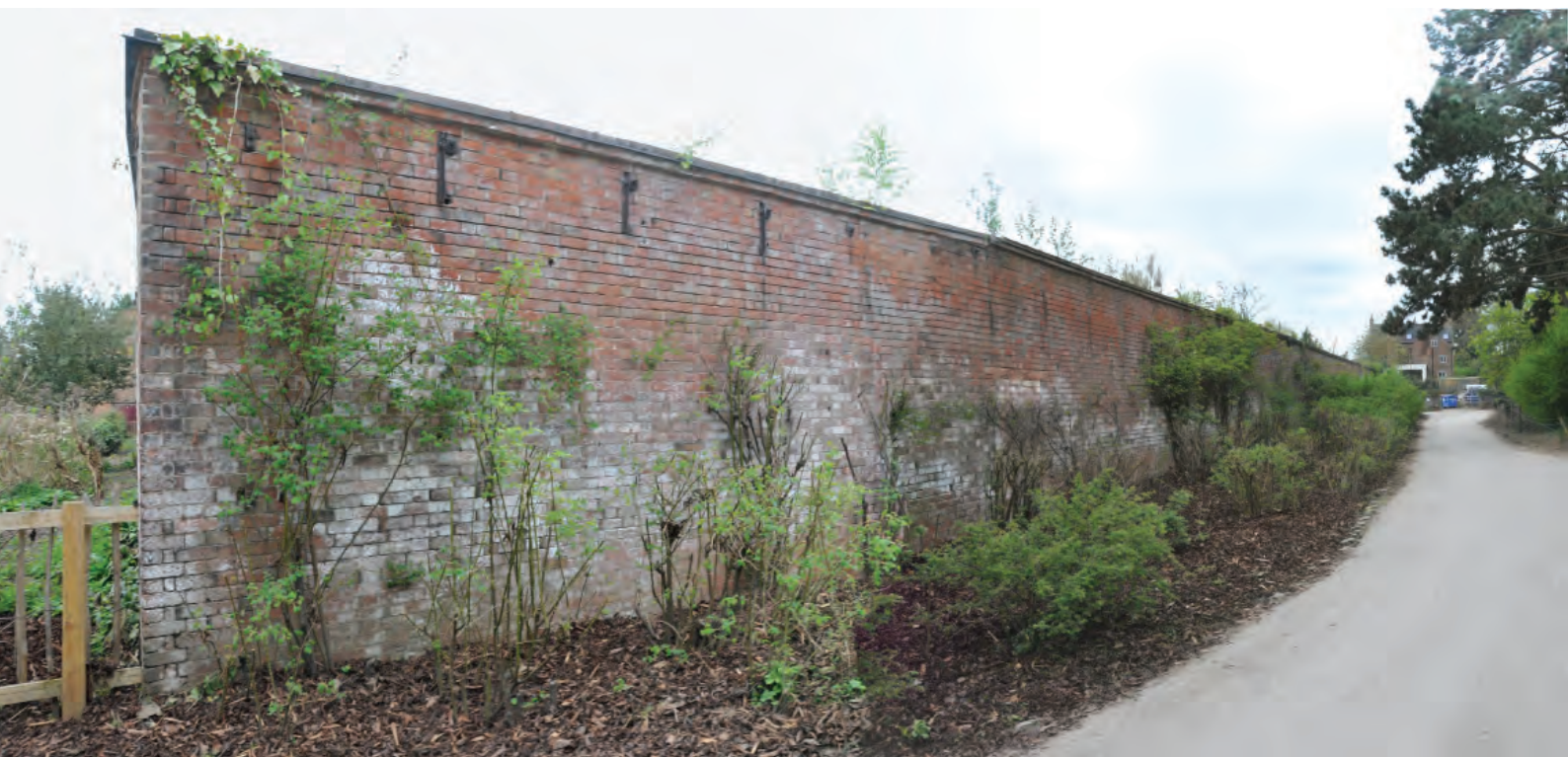
Fig. 6 (above): Panoramic view of north elevation of the heated wall; note the large format bricks used in comparison to those shown on; Fig. 7 (below): Panoramic view of west elevation of the former heated garden wall
