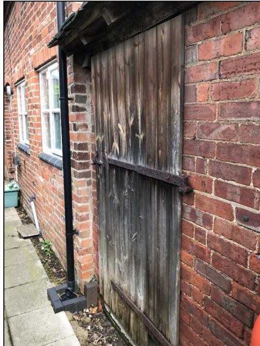
Plate 6. Door forming a void against the redbrick wall
