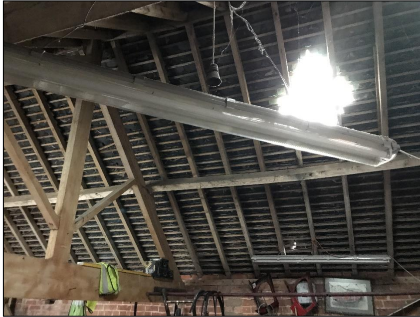
Plate 2. Roof structure and skylights located in barn one
