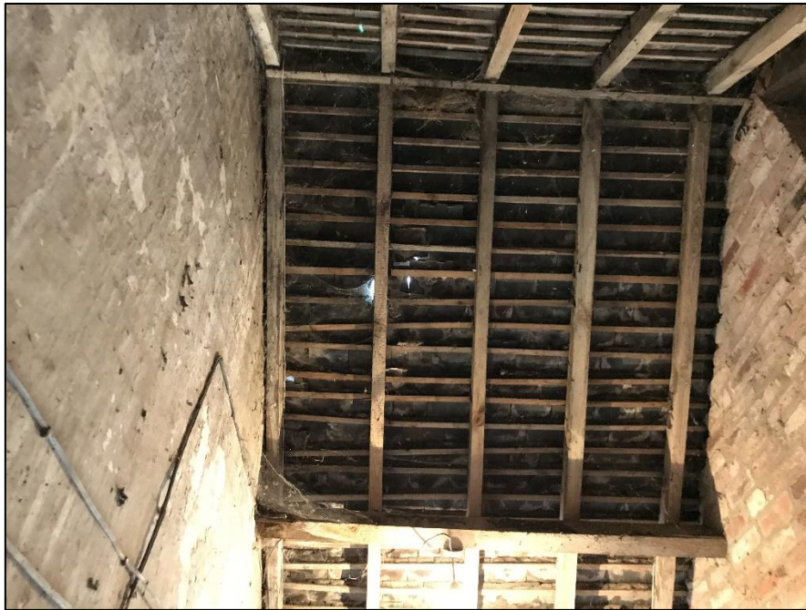
Plate 9. Roof structure and walls of the small storage space
