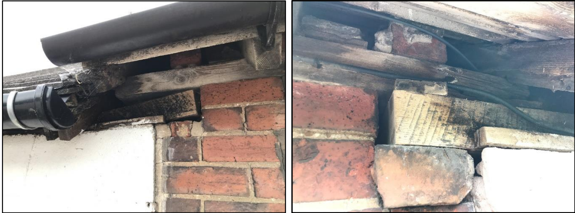
Plate 5. Suitable features located at the wall tops on the southern aspect of the building
