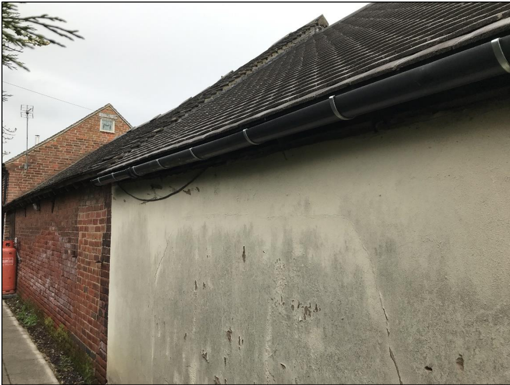
Plate 3. Southern Aspect of the buildings
