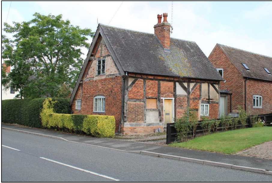
Plate 4.18: The Old Hall eastern and southern elevations
