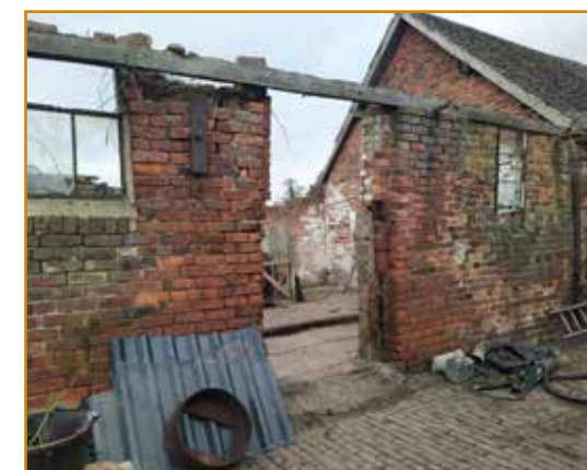
The proposed Utility doorway with the remaining gable of the Hall's ancillary wing behind
