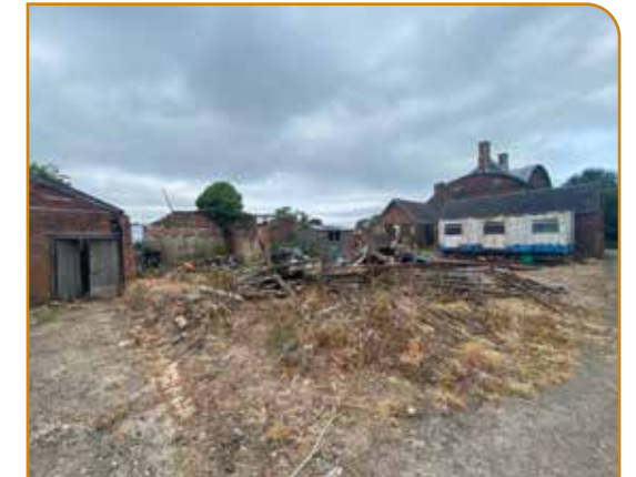
View of the site from the rear (south)—the proposed Games Room is on the left
