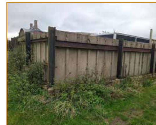
Existing boundary wall to be removed
