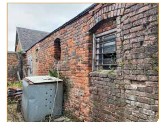
View of the remaining gable of the Hall's ancillary wing, showing the detached store in the foreground
