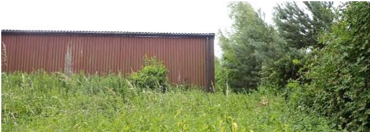
Photograph 3: North elevation of workshop, Riding Bank
