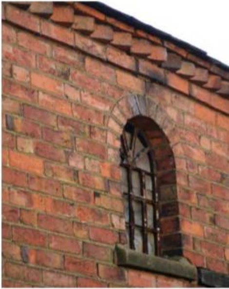
Above - corbelled sawtooth brick eaves and semi-circular arched cast-iron window at 7 Derby Rd.
