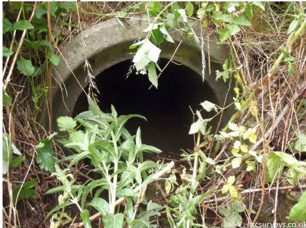
Upstream face, looking downstream
