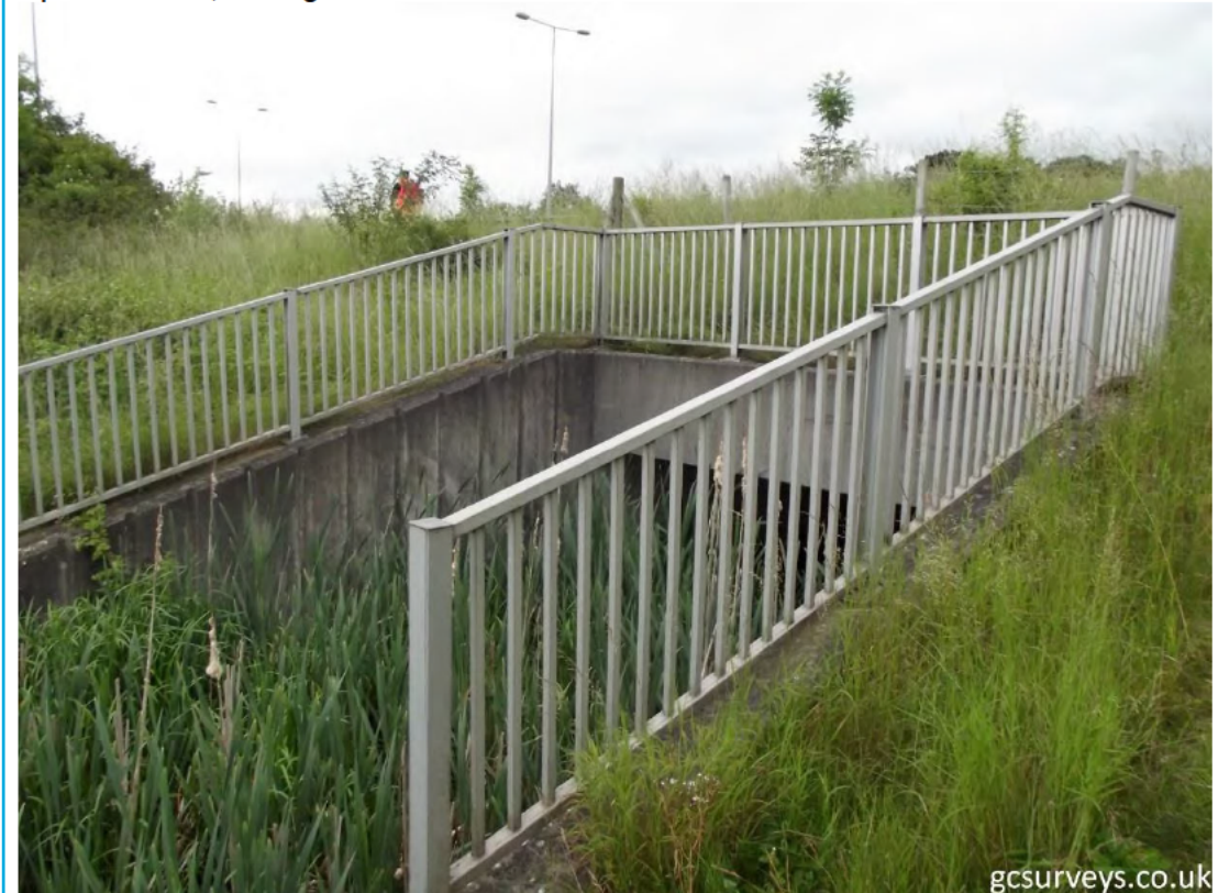
Upstream face, looking downstream
