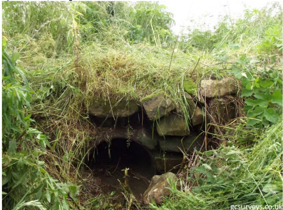
Upstream face, looking downstream
