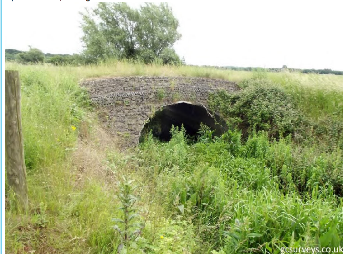
Upstream face, looking downstream
