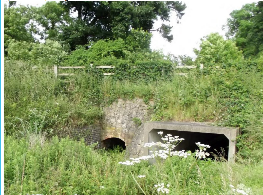
Upstream face, looking downstream
