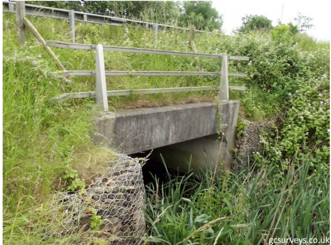
Upstream face, looking downstream
