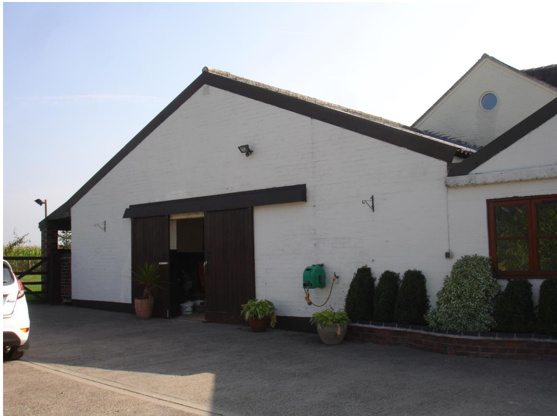
View from west of North barn
