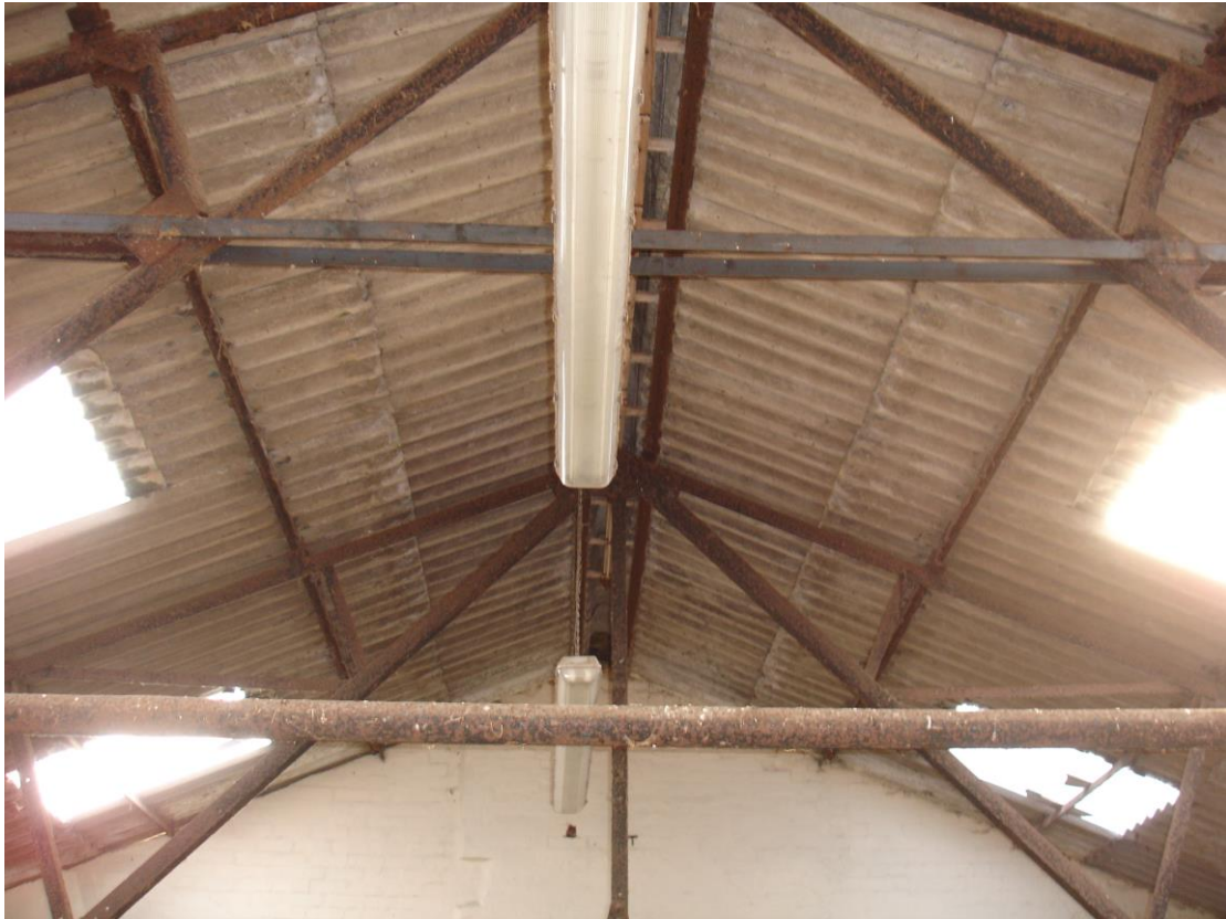
View looking east
