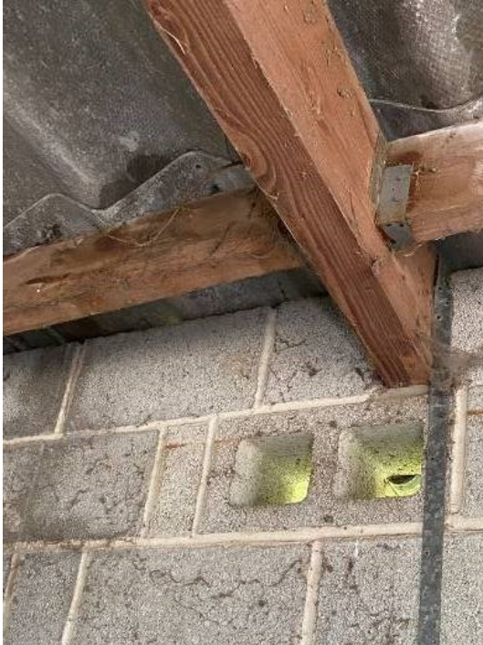
Figure – primary beam penetrating front wall with restraint strap and incoming purlins
