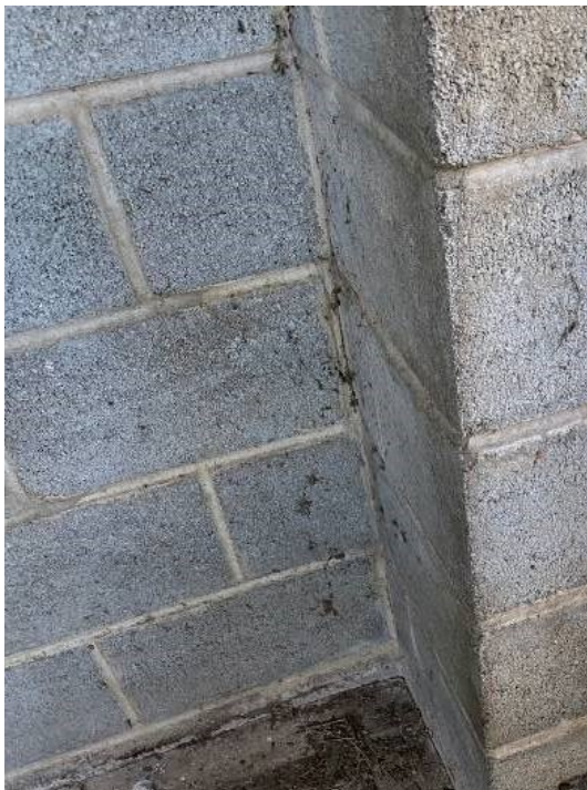
Figure – floor slab cast within masonry walls – not off.
