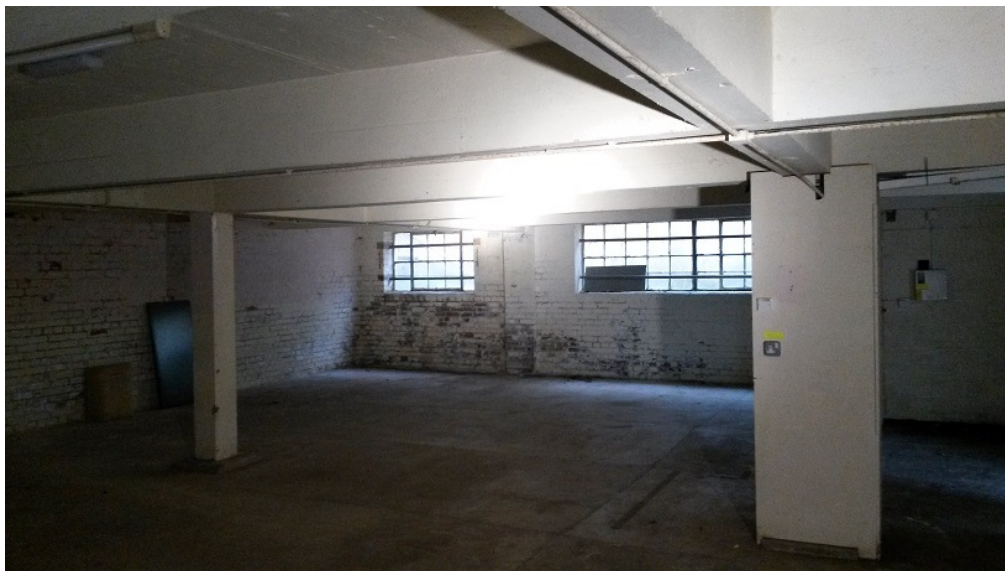
Photo: Basement leading to rear loading bay
