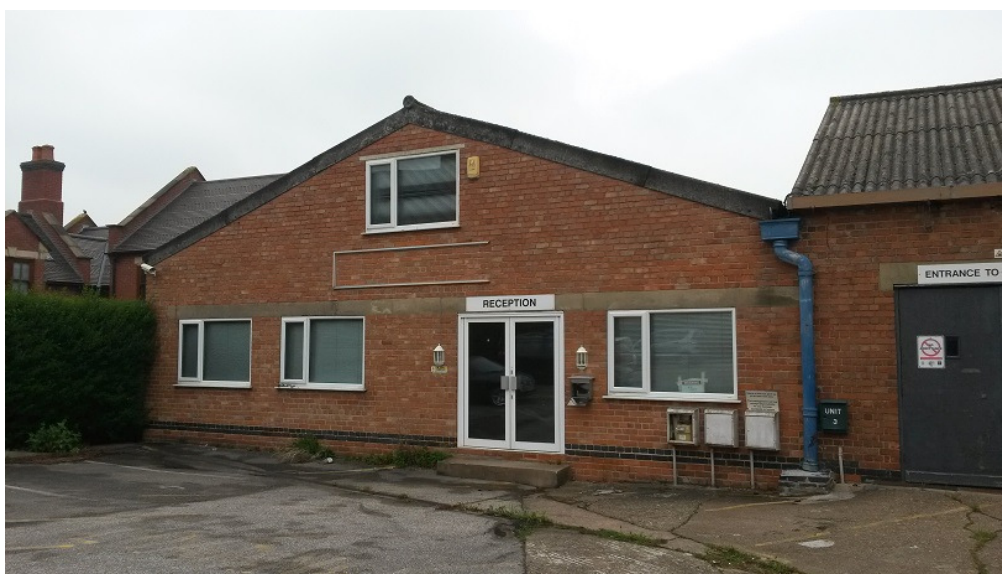
Photo: Front of office building B2
