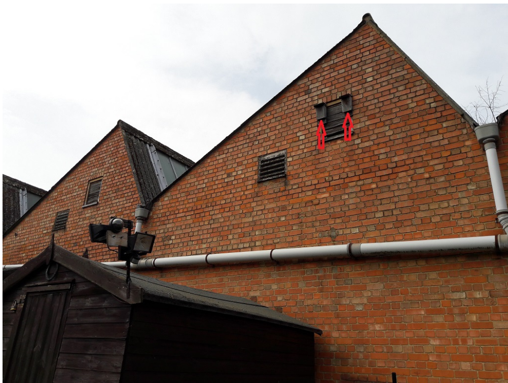
Photo: Wooden bat boxes on eastern wall of B1
