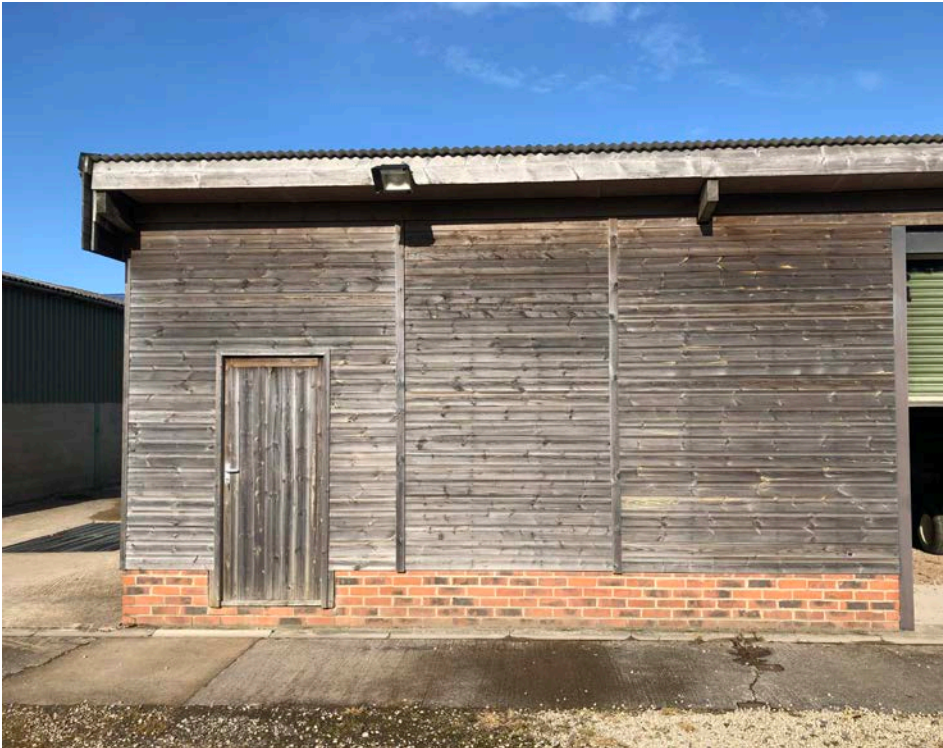
12. Front (east) elevation of timber office storage shed
