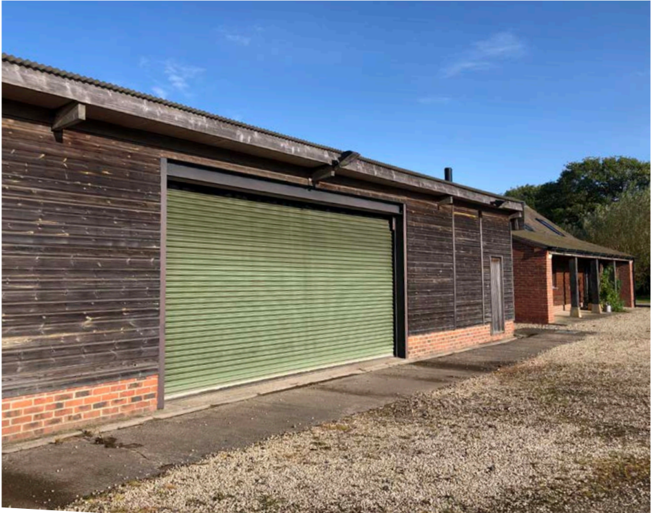
5. East elevation of timber office storage shed and red brick boiler house beyond
