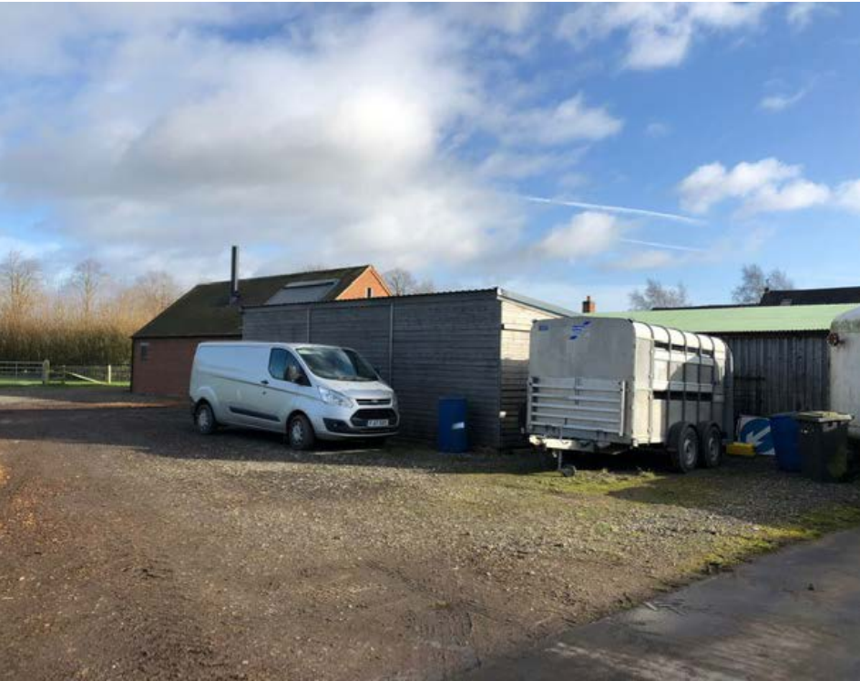
11. Rear of timber office storage shed and red brick boiler house
