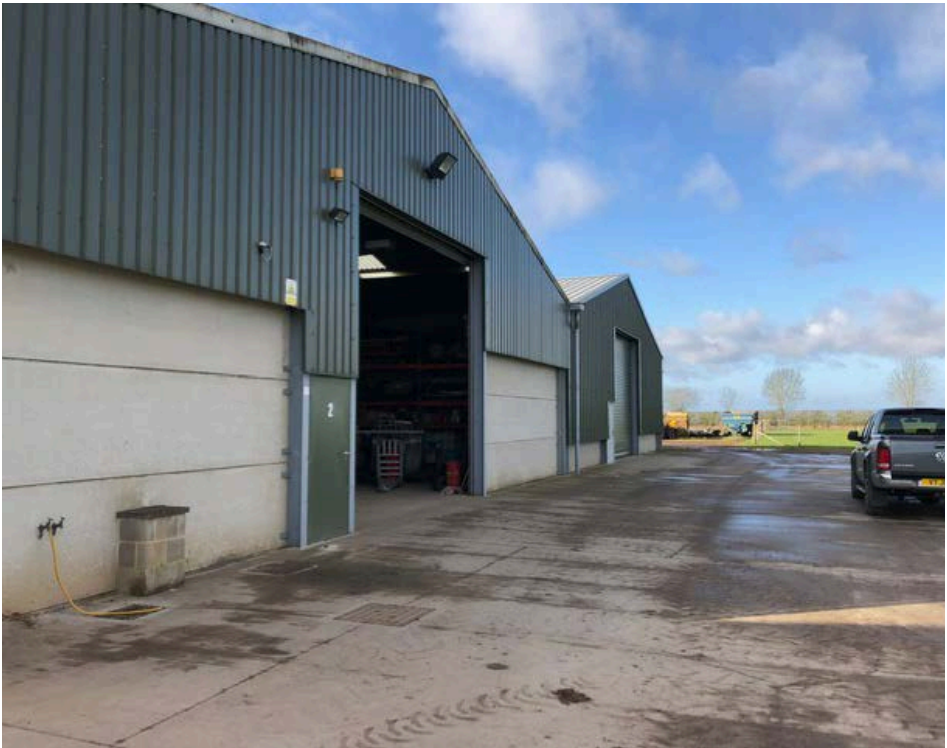
2. Northern elevation of agricultural sheds 2 and 3 on site
