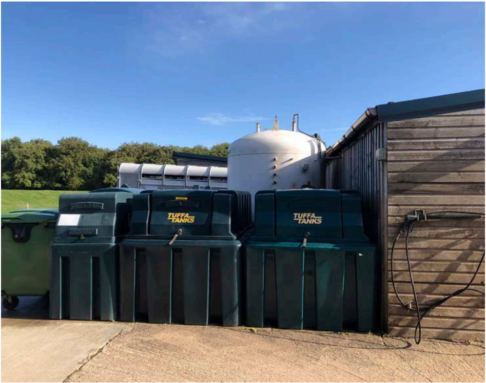
13. View of side and rear of timber office storage shed looking north
