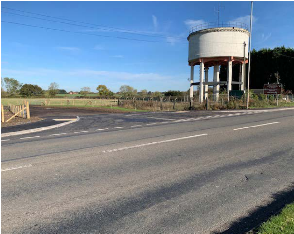
View of newly constructed access road from Ashby Road
