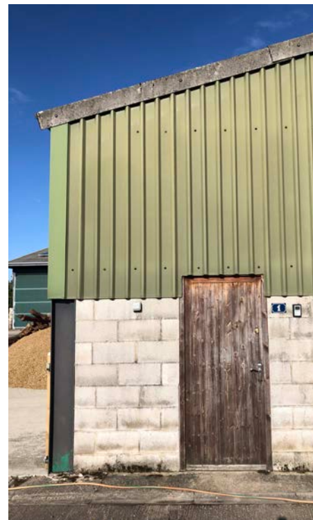
7. East elevation of metal clad, blockwork walls and steel portal frame agricultural shed
