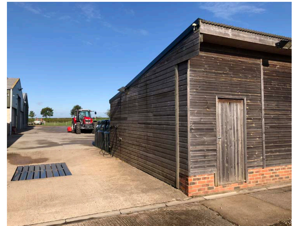
8. South elevation of timber office storage shed looking north west
