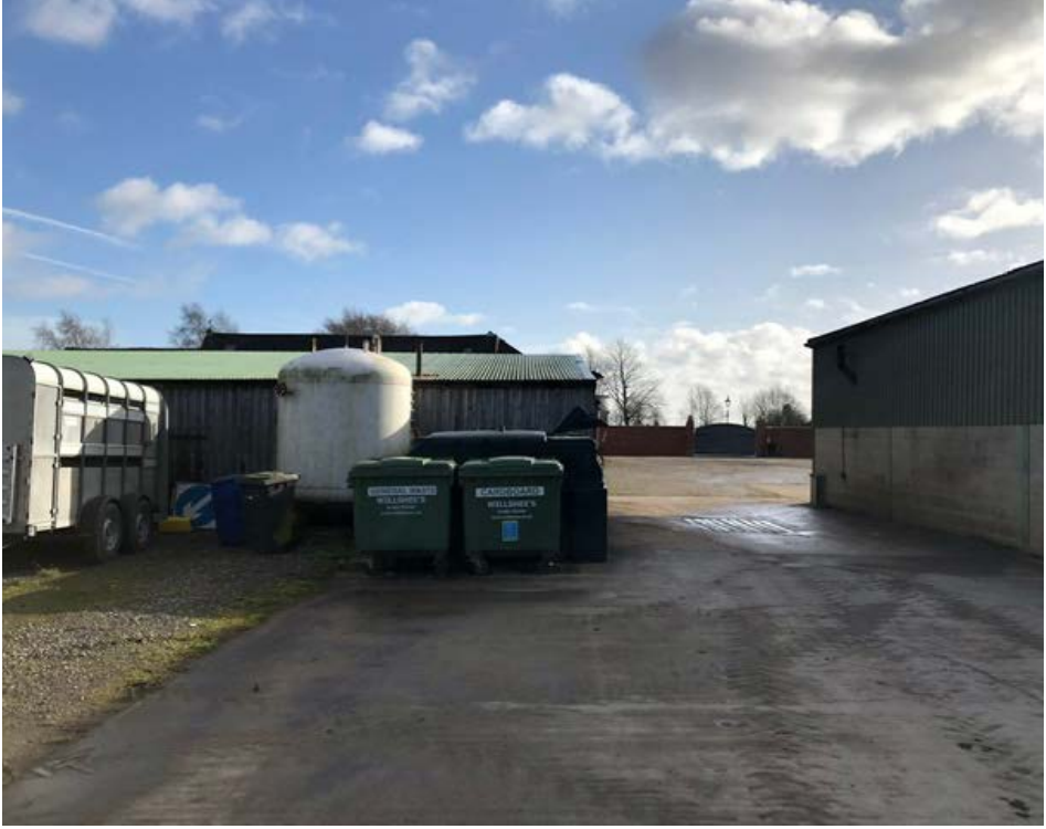
16. Rear (west) elevation of timber agricultural shed looking east
