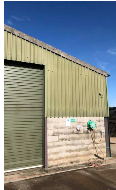
7. East elevation of metal clad, blockwork walls and steel portal frame agricultural shed
