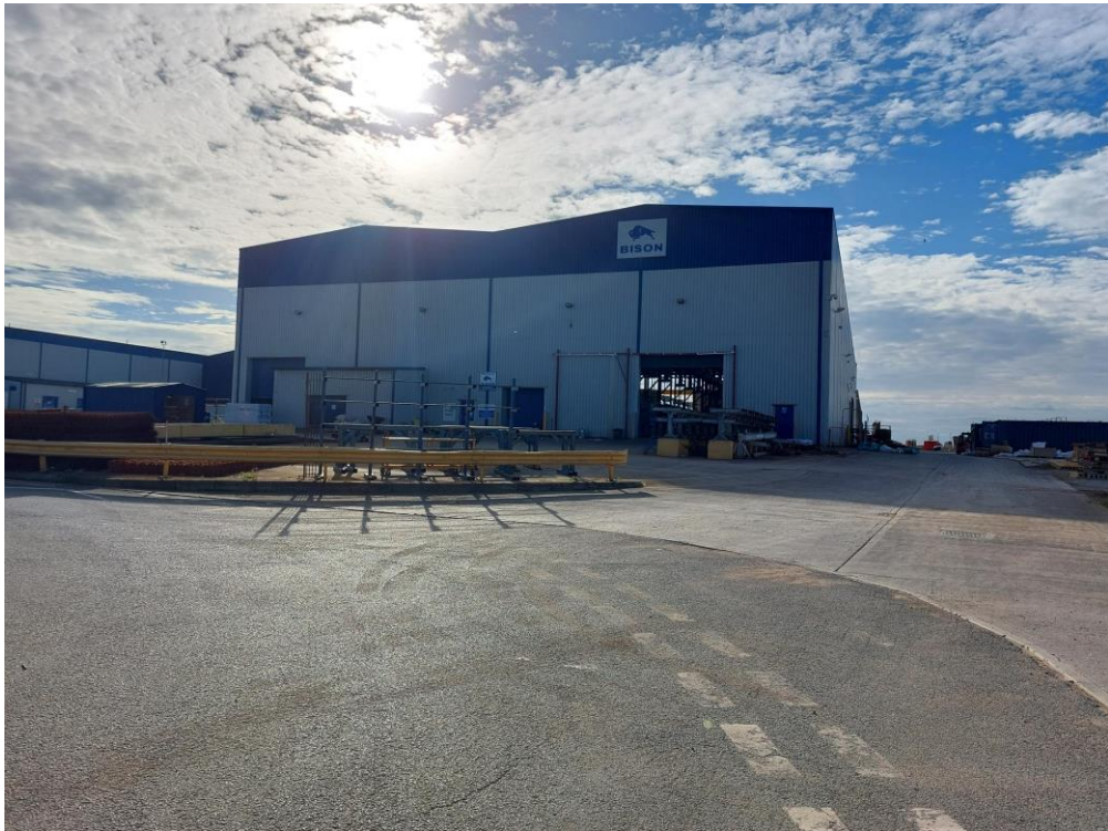
Plate 4. Metal buildings for demolition
