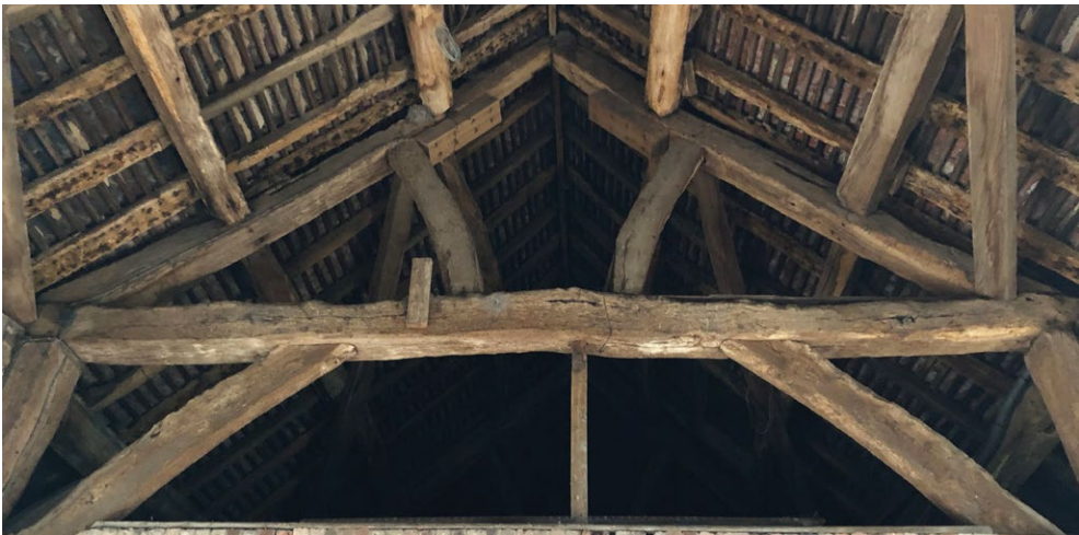
Fig.11 Existing cross frame with queens post trusses
