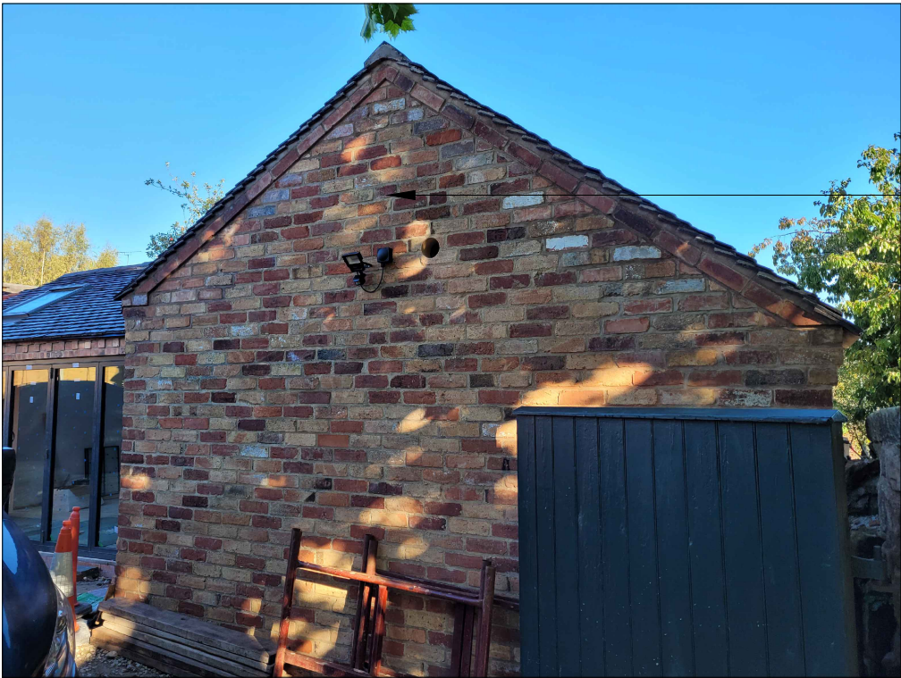
South Elevation (Illustrating brick corbel Eaves detail)
