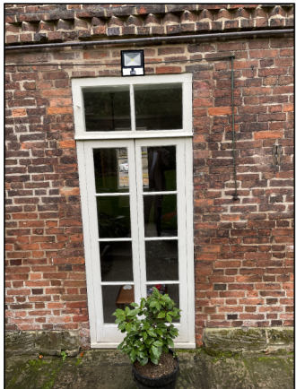
View of patio doors with PIR Light over.
