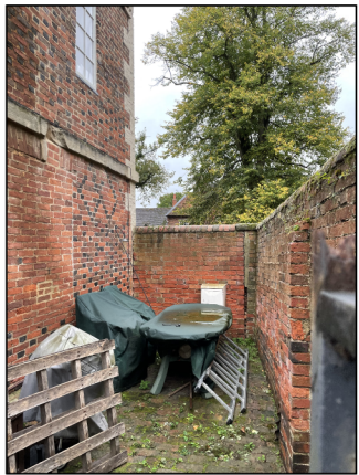
View of side area
