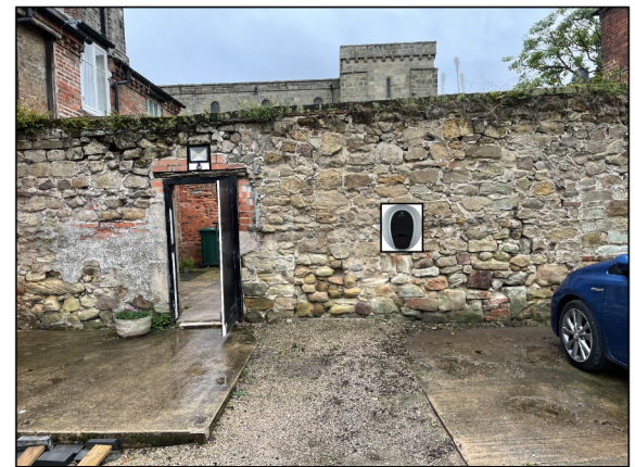
View of existing wall with proposed charging point and light
