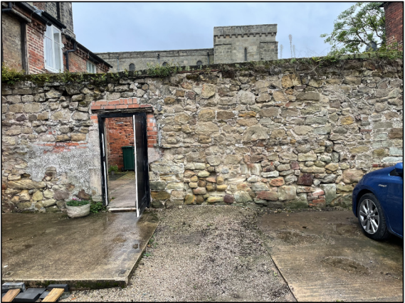
View of existing wall
