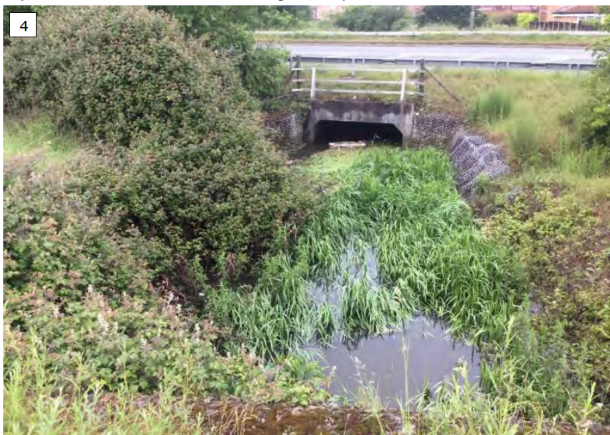
Figure 2-4: Particularly over-wide channel within the vicinity of the culverts
