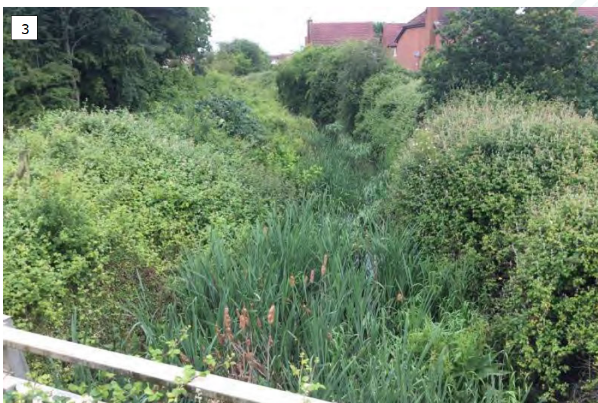
Figure 2-3: Thulston Brook looking upstream from Chellaston Lane
