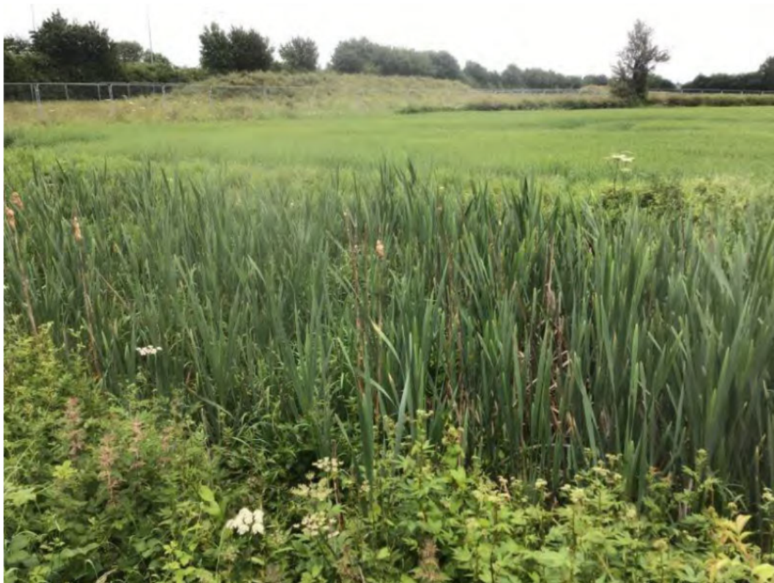
Figure 3-1: Thulston Brook at the eastern perimeter of the site. Here the channel is choked with emergent vegetation.
