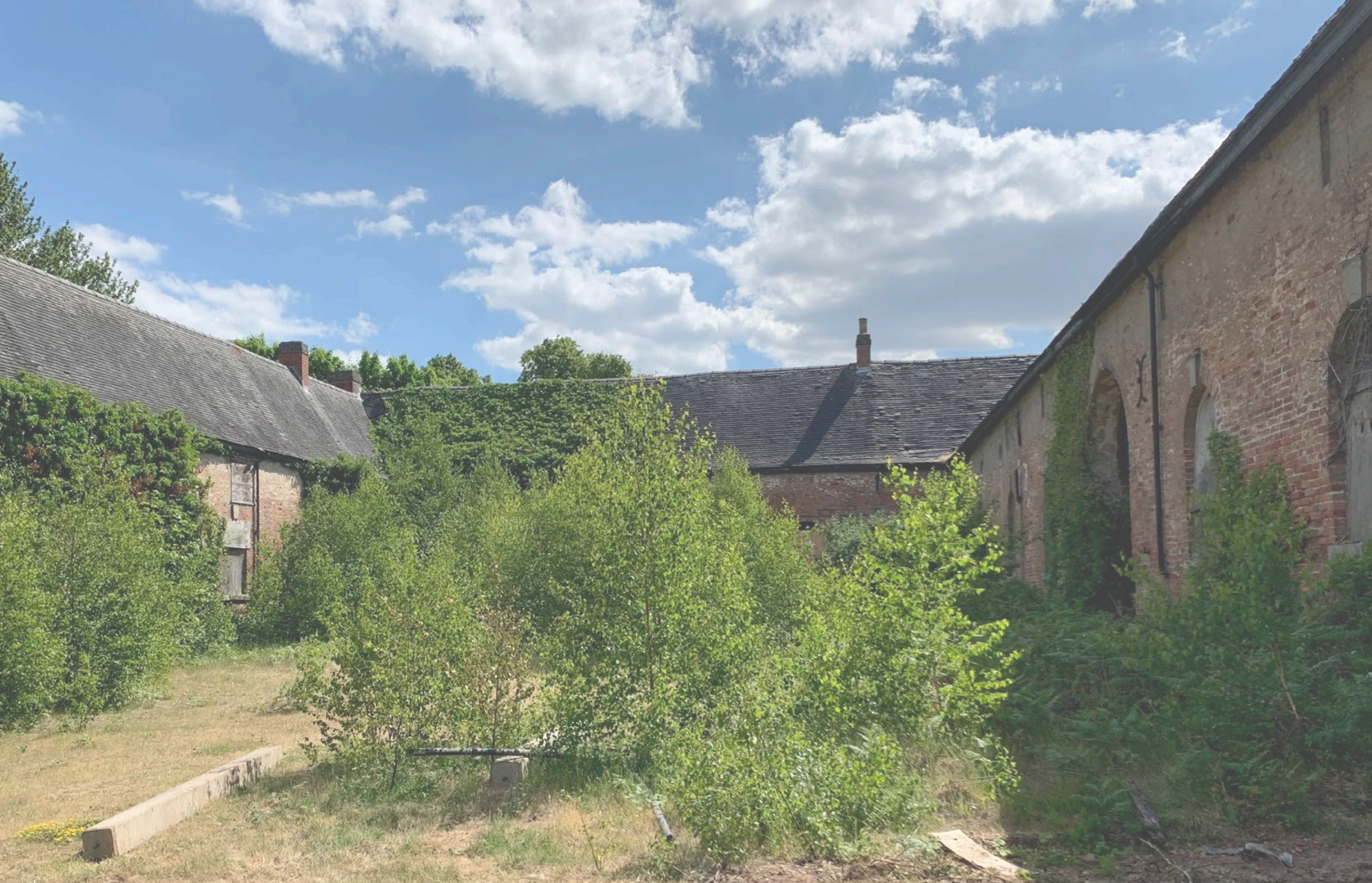
THE APPLICATION SITE
