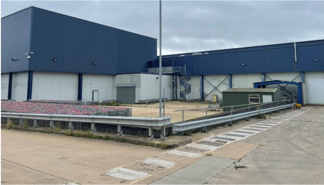
Figure 2.3 – The Site viewed from the north west, looking south east
