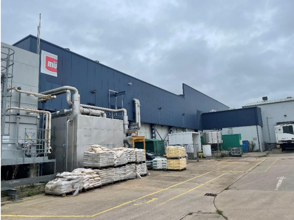
Figure 3.2 – Proposed location for the extension to the southern elevation. Viewed looking north east towards the southern elevation from the south western corner of the site
