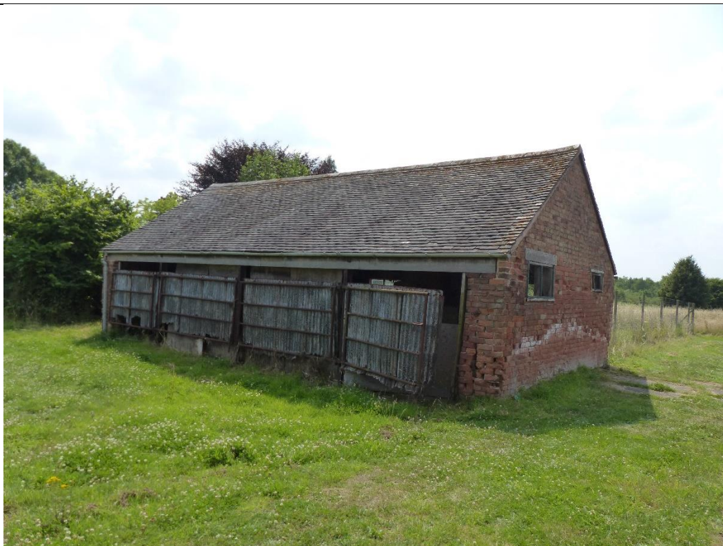
Photo 2 - General view of Barn 2 - Elevation B1
