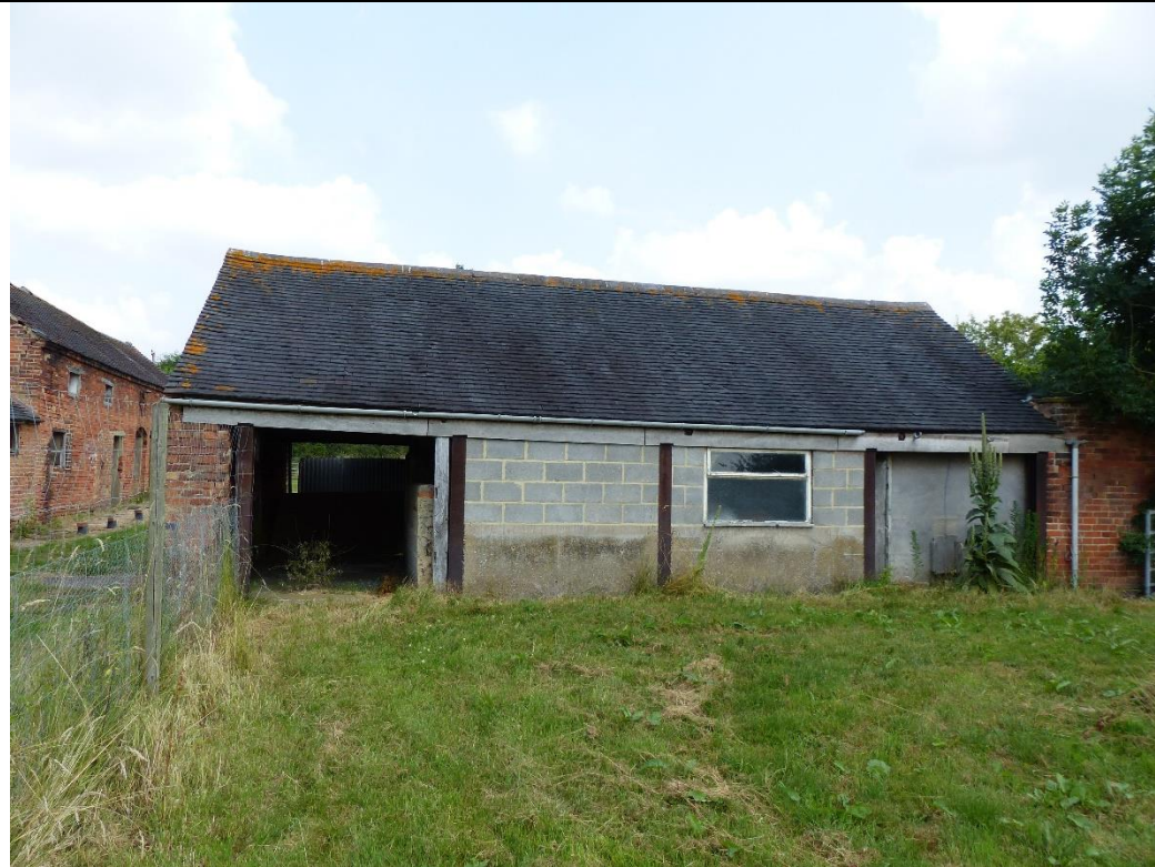
Photo 11 – Barn 2 – Blockwork infill sections
