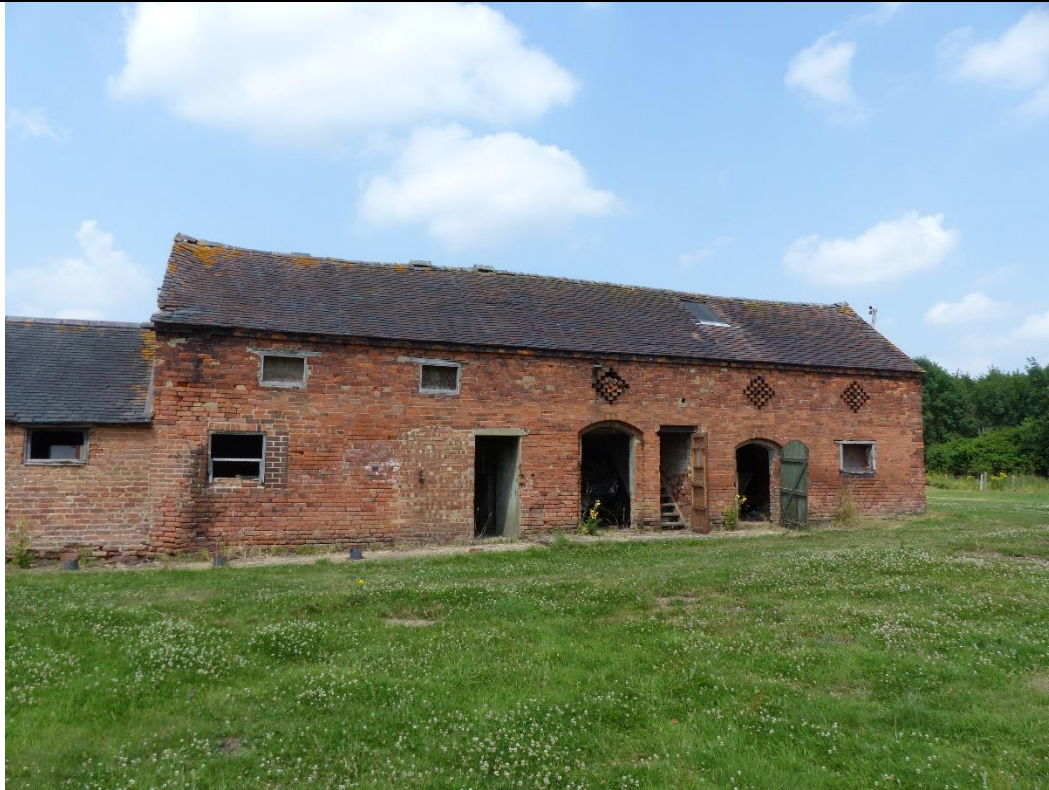
Photo 1 - General view of Barn 1 - Elevation A1
