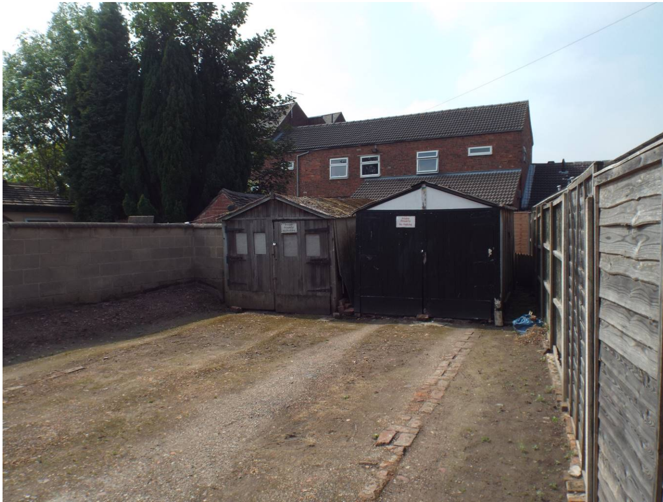
Garages to be demolished
