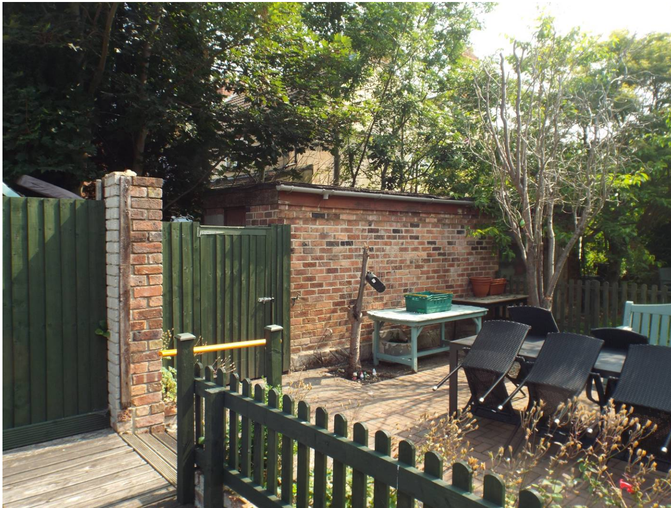
Outbuilding converted to laundry
