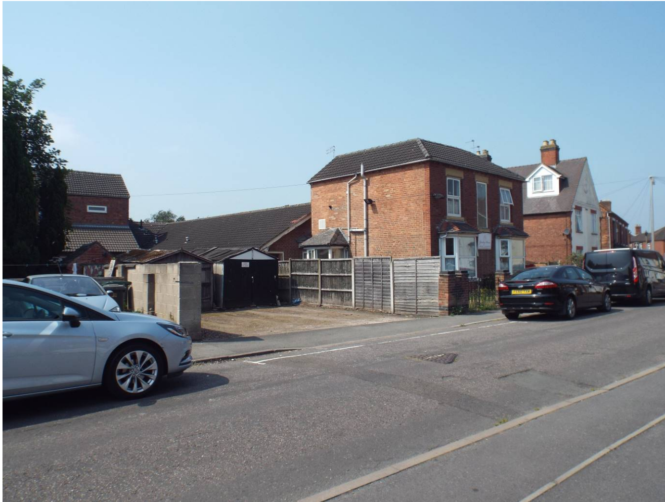
Existing building extended towards left
