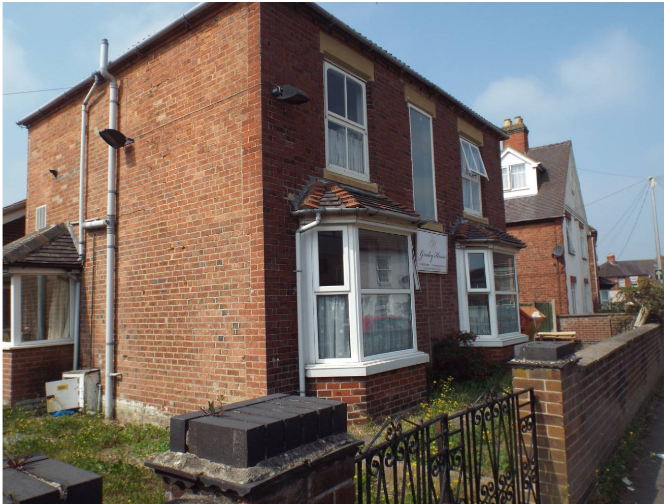
Existing building to be extended
