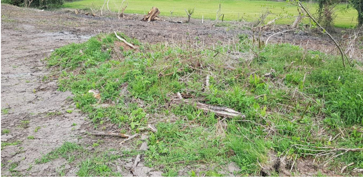
Photo 15. Remains of brick-built septic tank cesspit.
