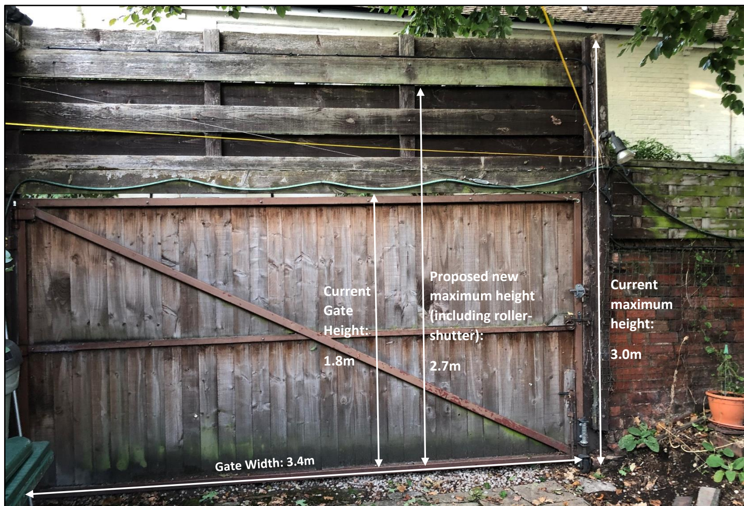
Figure 5: Close-up of gate to be replaced
