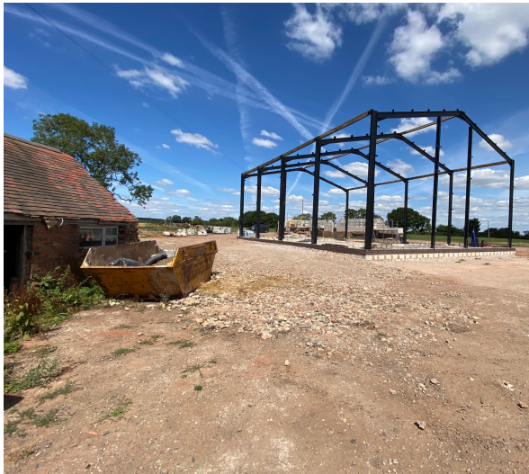
Image 1: B6 left in-situ at left corner of the image. New building under construction in main frame of image
