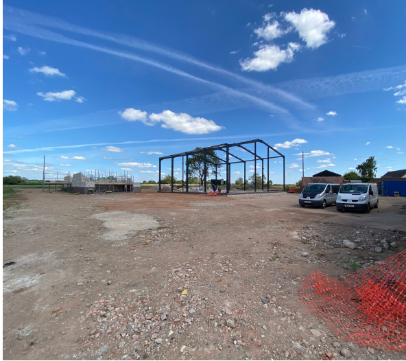
Image 5: New buildings under construction, looking in a north-easterly direction
