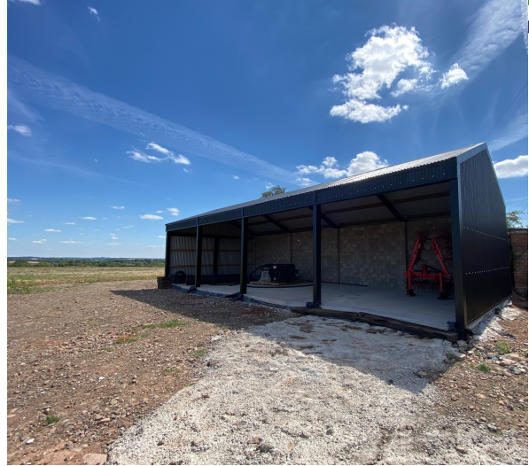
Image 6: Recent building construction positioned beyond existing red line boundary marked in previous reports. Looking in an easterly direction
