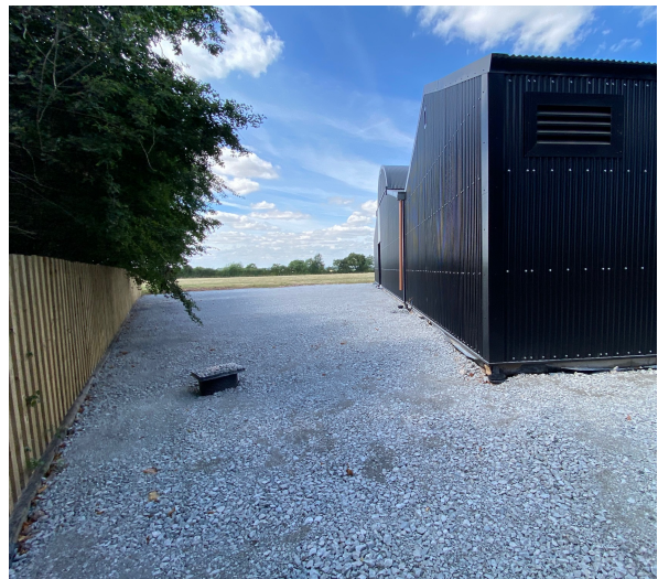
Image 4: Hard compacted habitat at southern boundary, looking in a westerly direction
