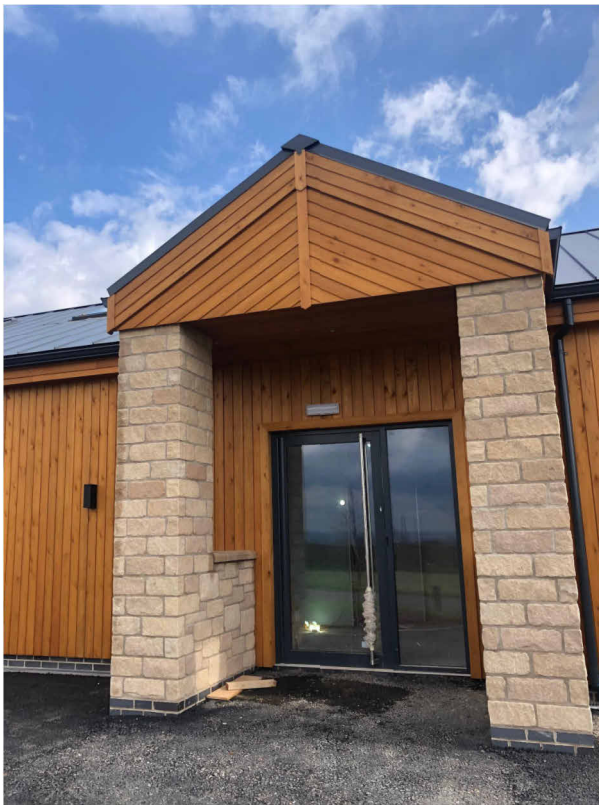
STONE PORCH - AS CONSTRUCTED
